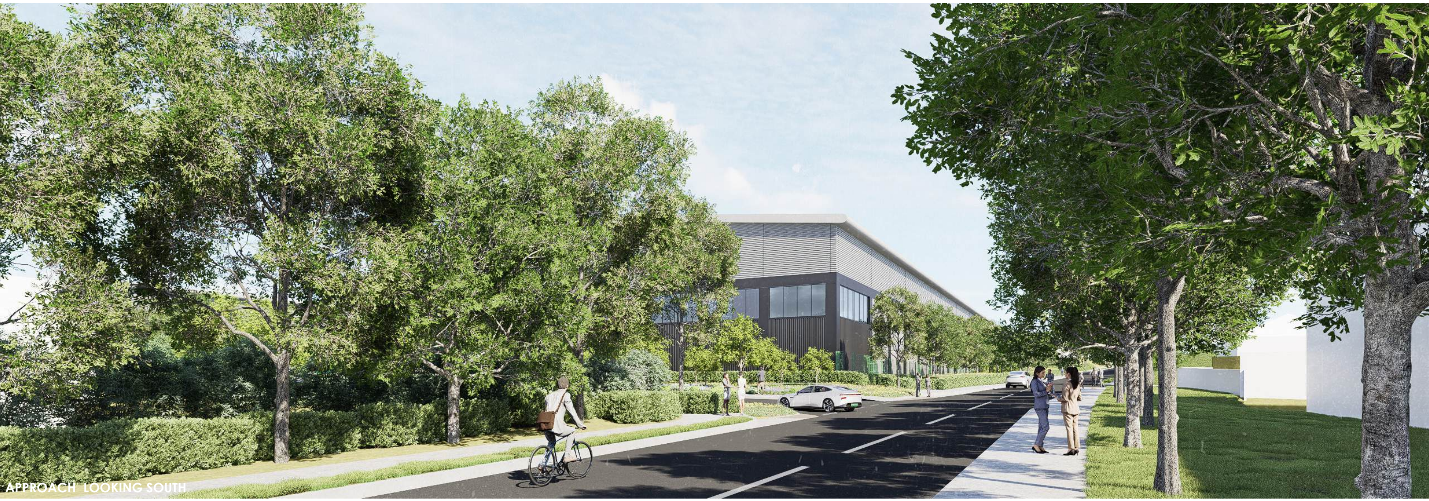
APPROACH LOOKING SOUTH
