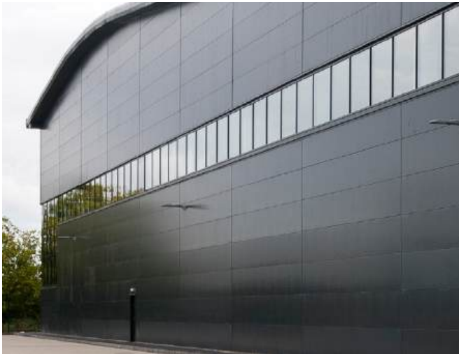
FLAT PANEL CLADDING TO ACTIVE ELEMENTS OF THE BUILDINGS
