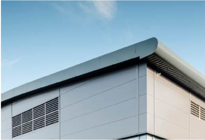
CURVED ROOF WITH EXPRESSED OVERHANGS
