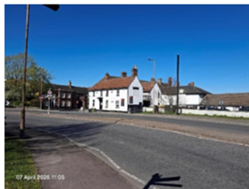
Context image, taken from the A10, majority of the former unauthorised signage removed. One piece attached to the gable end remains.
