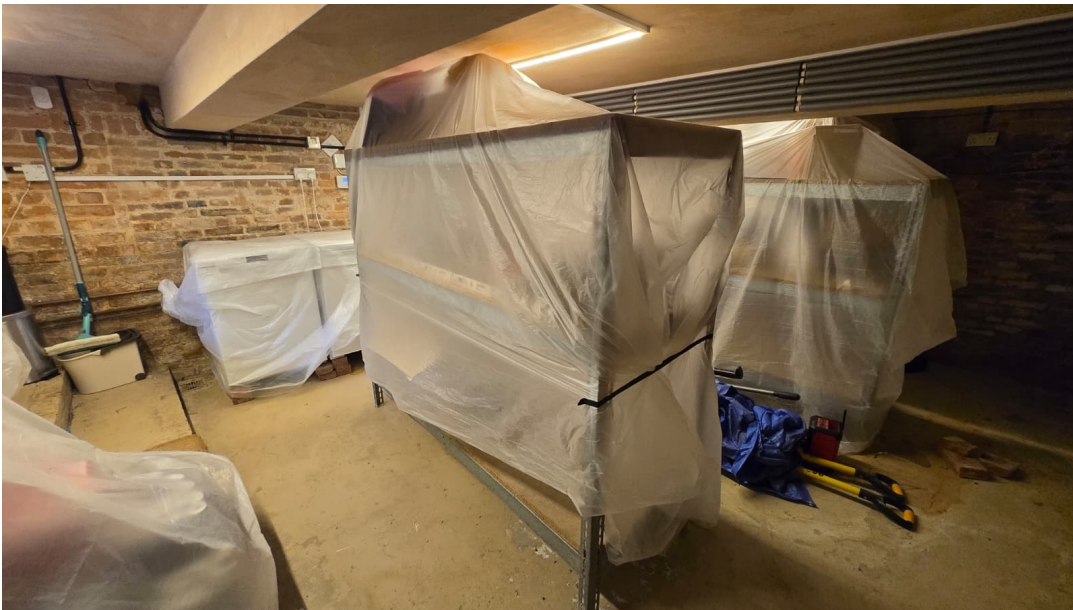
contemporary photo of cellar
