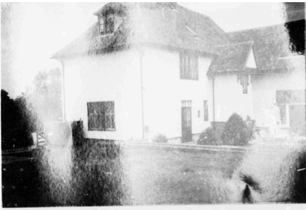
historic photo of west wall (prior to addition of garden room c.2000)
