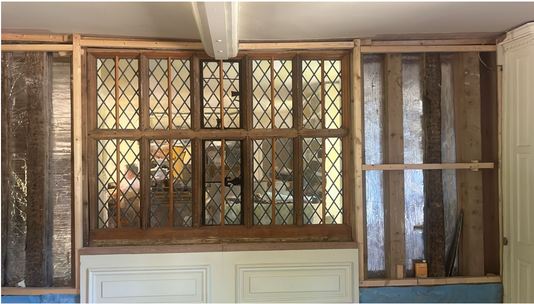
contemporary internal photo of existing window in west wall
