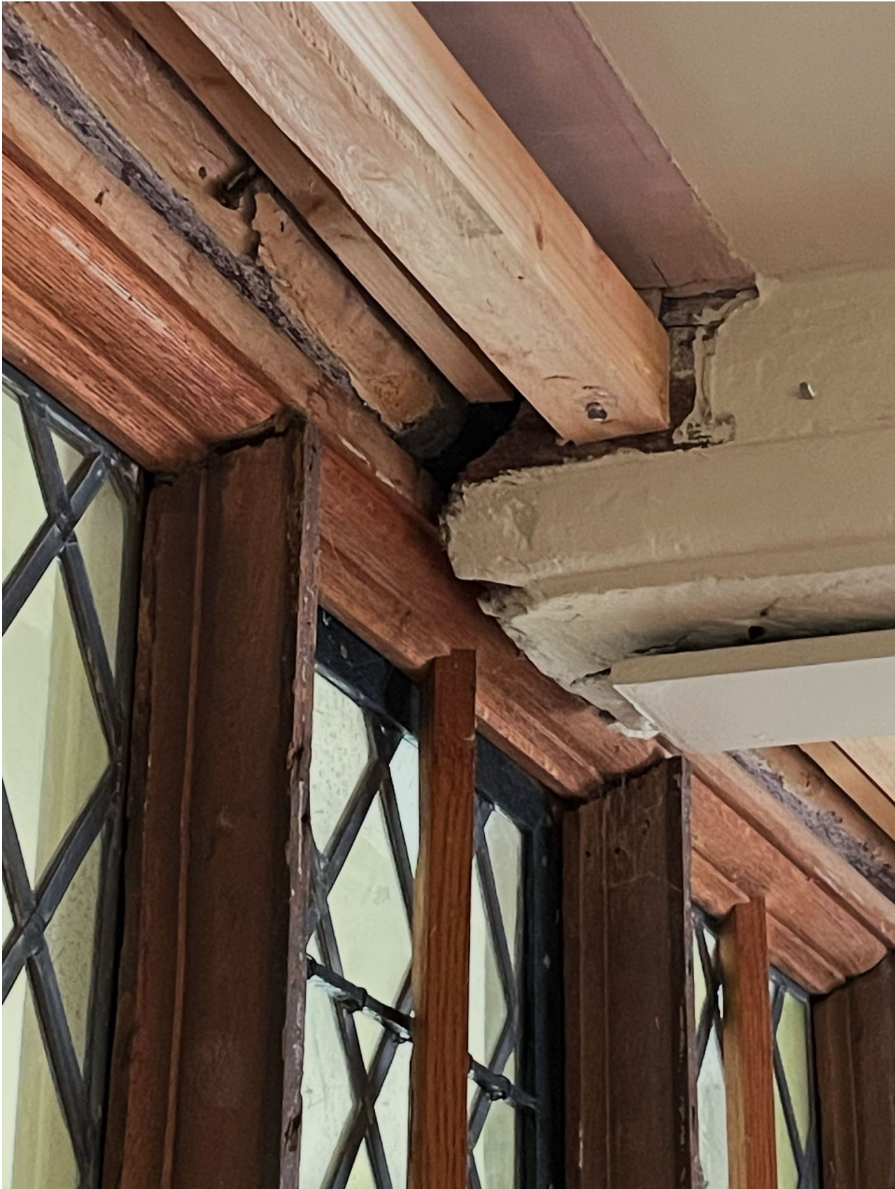
BEARING ONTO EXISTING WINDOW FRAME
