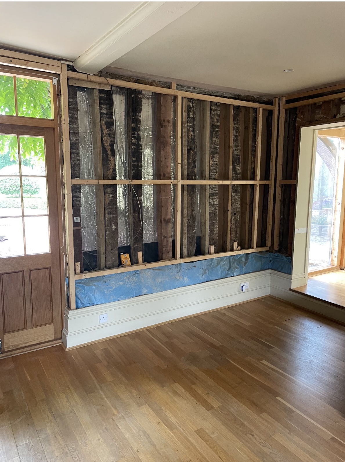
GROUND FLOOR DINING ROOM SHOWING END BEARING OF SECONDARY TIMBER SUPPORT
