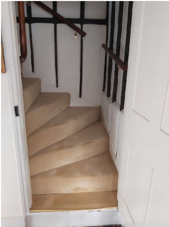
Step at bottom of internal staircase creating low head clearance, necessitating extension to accommodate stair lift
