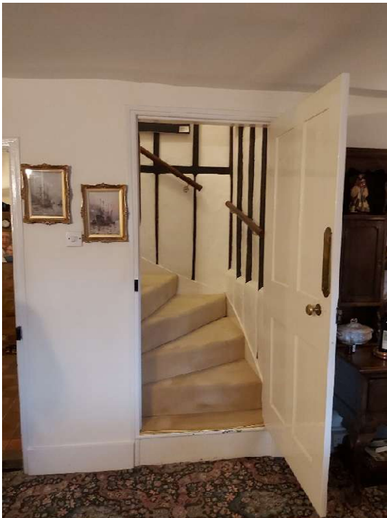
Step at bottom of internal staircase creating low head clearance, necessitating extension to accommodate stair lift
