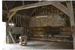
Figure 39: Internal of store- note the brick infill in the gable end
