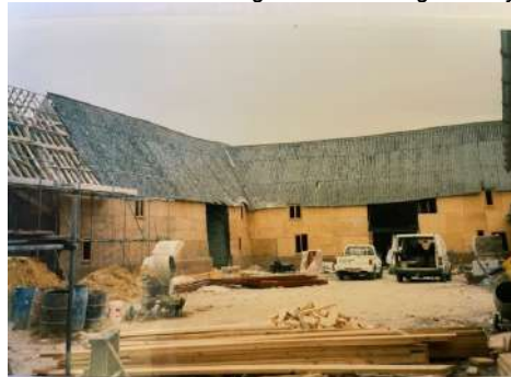
Daubentons Barn with the timber frame bracing being added and openings appearing.
