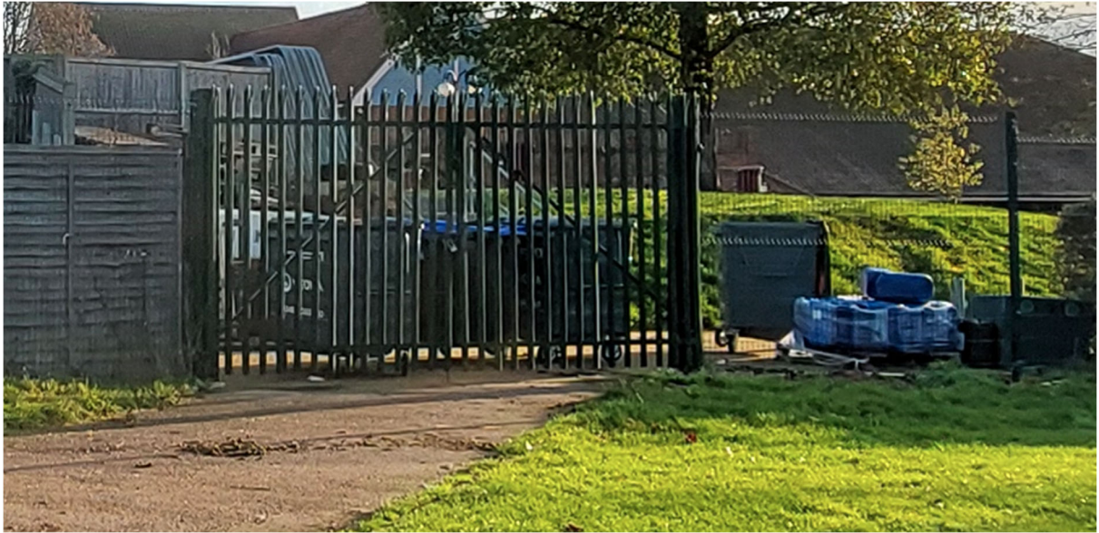
Existing Palisade gate (green)
