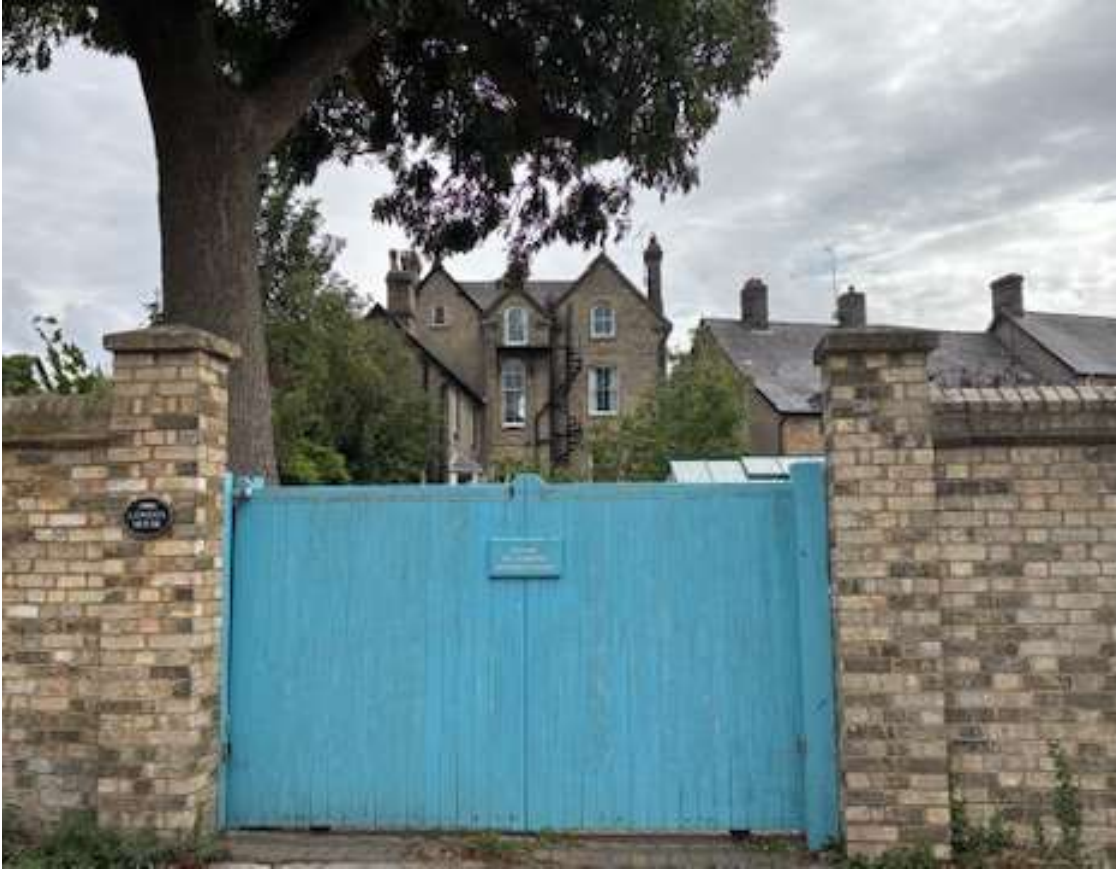
Photo 8 – Rear entrance & elevation viewed from Hodwell
