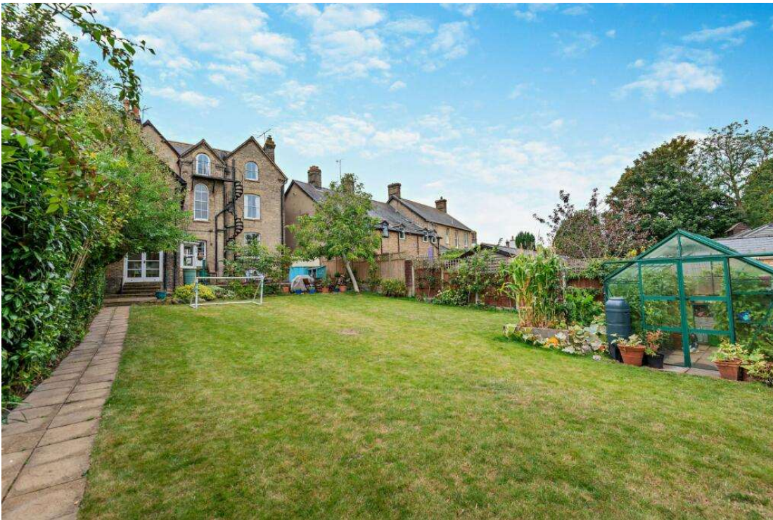
Photo 7 – Rear Elevation viewed from further down the garden
