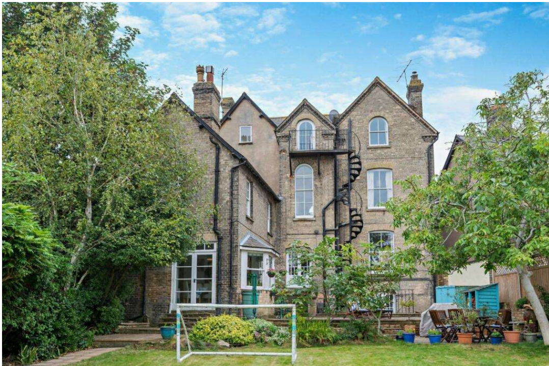
Photo 2 – Rear Elevation and patio viewed from the garden
