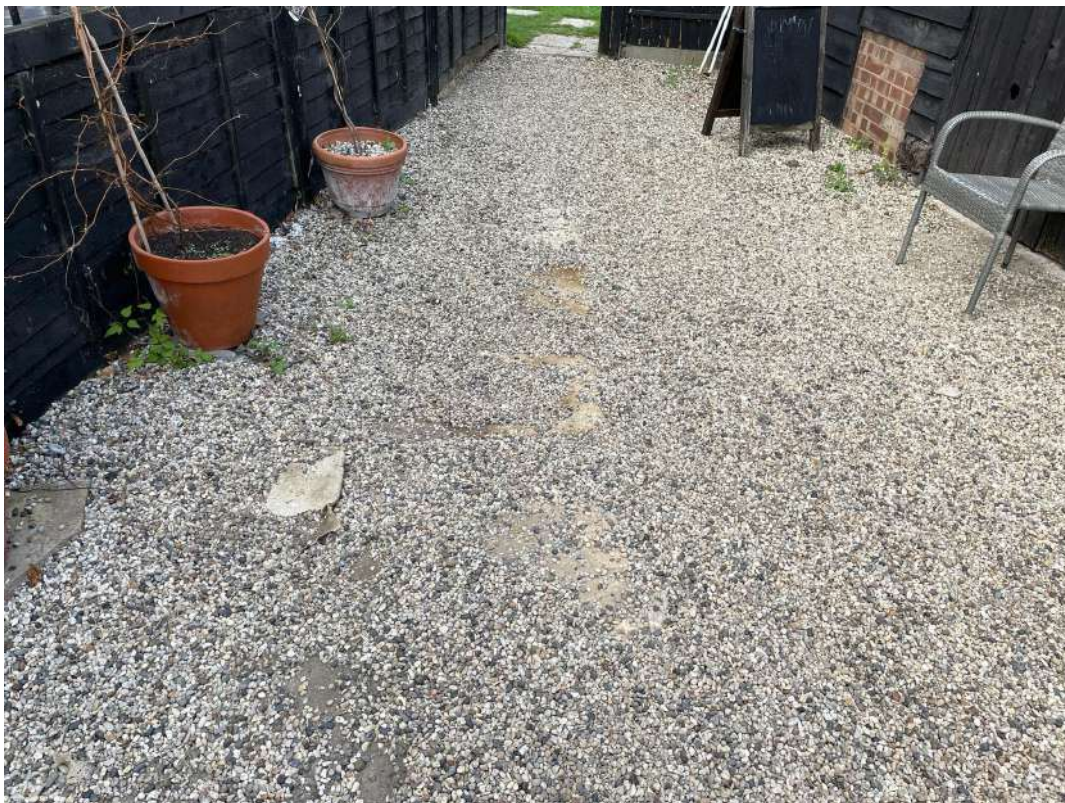
Photograph 8: View west showing concrete foundations of possible former structure.
