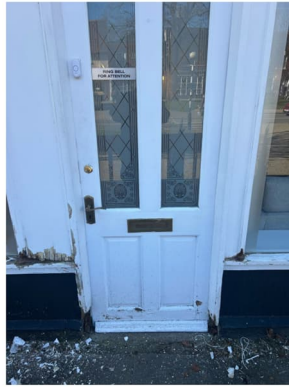
Existing Door Condition
