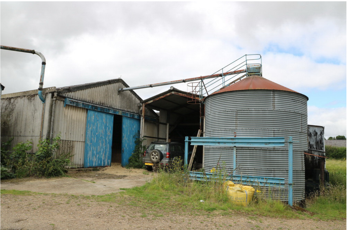
Plate 10 - Grain silo in angle between Barns 2a & 2b, facing SW
