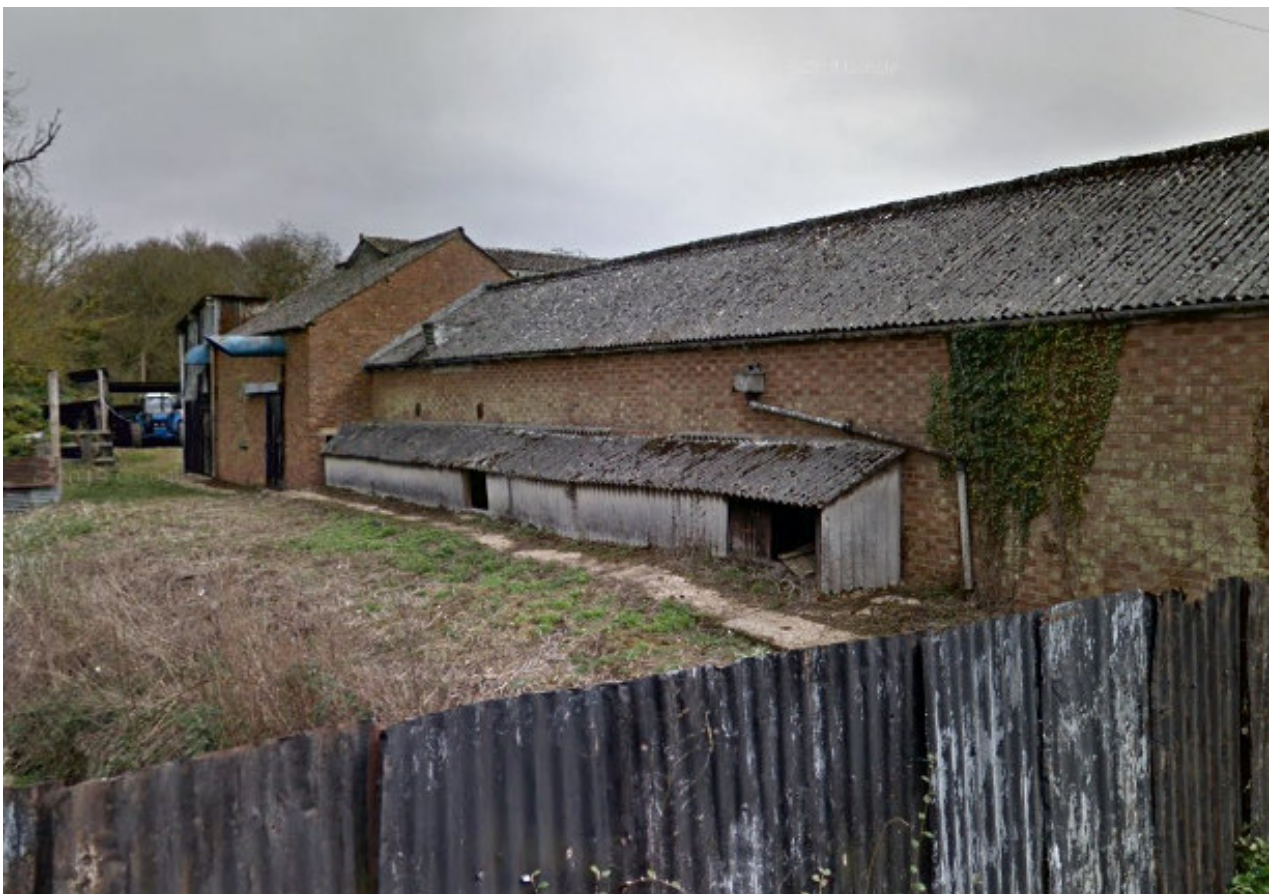
Plate 02 - Lean-to carrying duct alongside Barn 1, facing NE (Courtesy Google Streetview)
