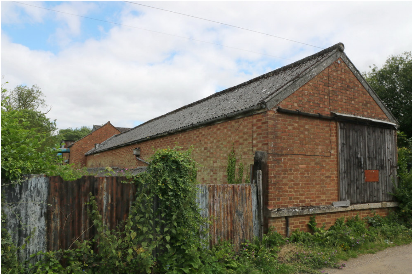
Plate 01 - Barn 1, south & west elevations, facing NE
