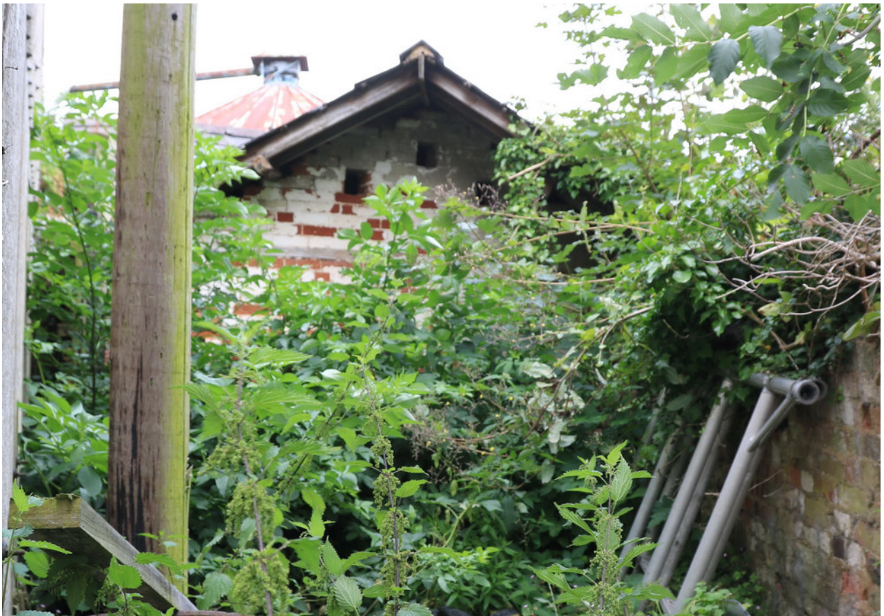
Plate 08 - Barn 4, south elevation, facing N
