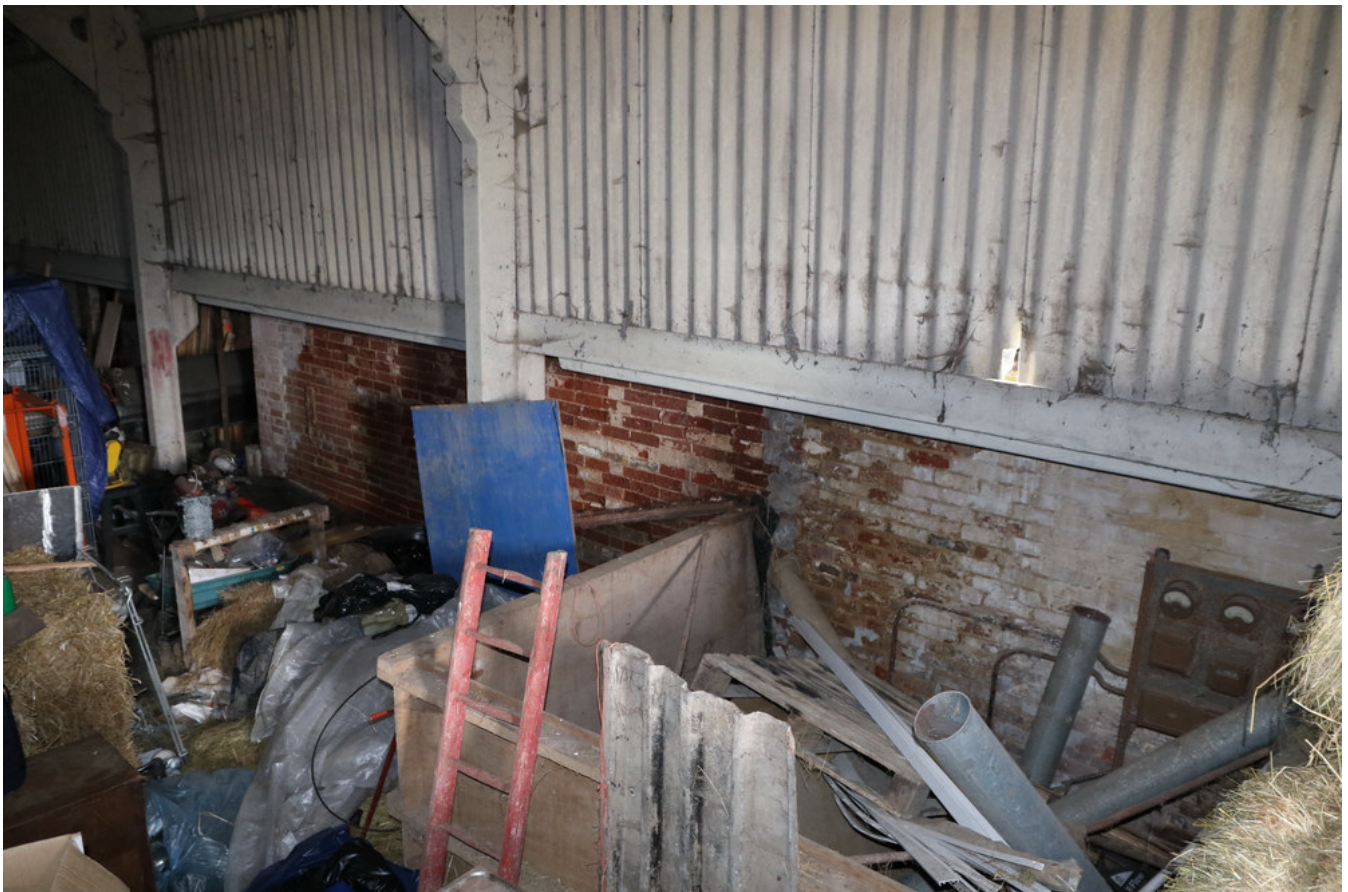
Plate 12 - Earlier brickwork in east elevation of Barn 1, facing SW
