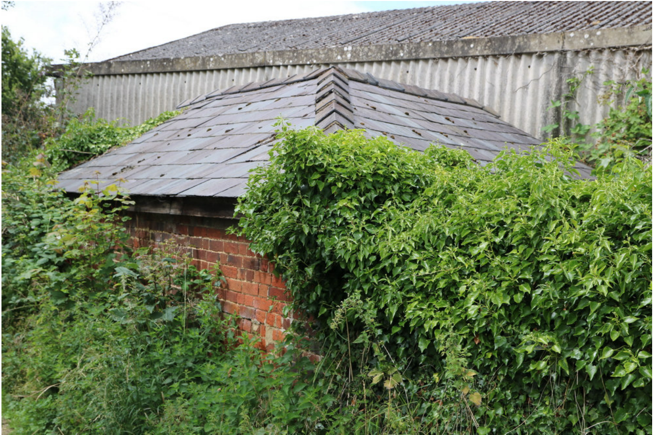
Plate 07 - Barn 4, facing SW
