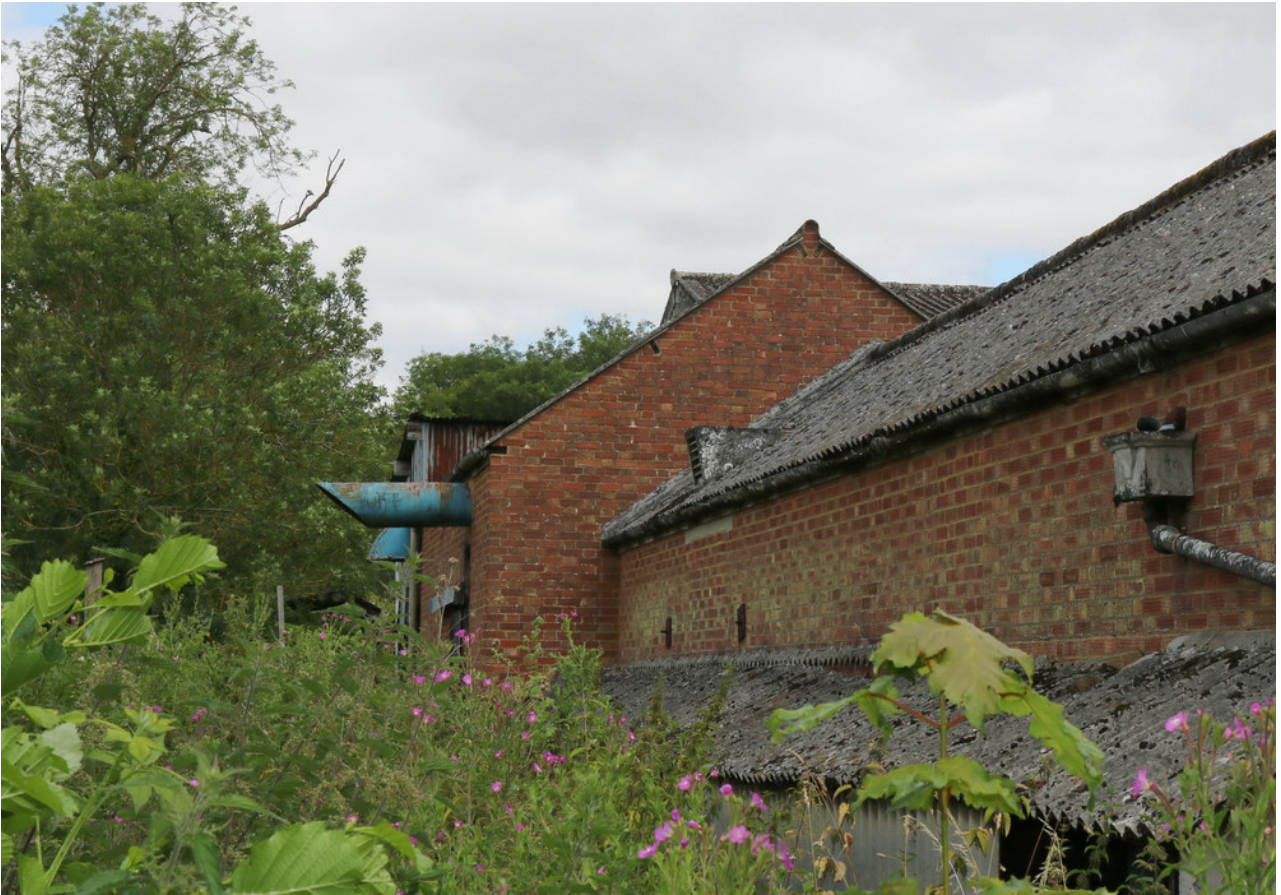
Plate 03 - Barn 2, south and west elevations, facing NE
