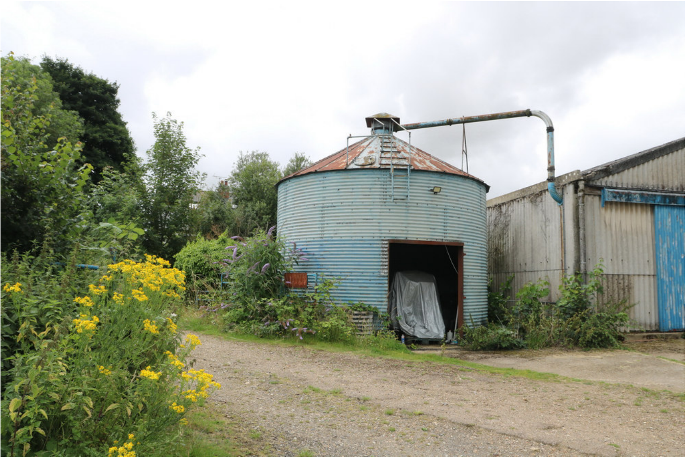
Plate 09 - Grain silo in N angle of Barns 3 & 4, facing S
