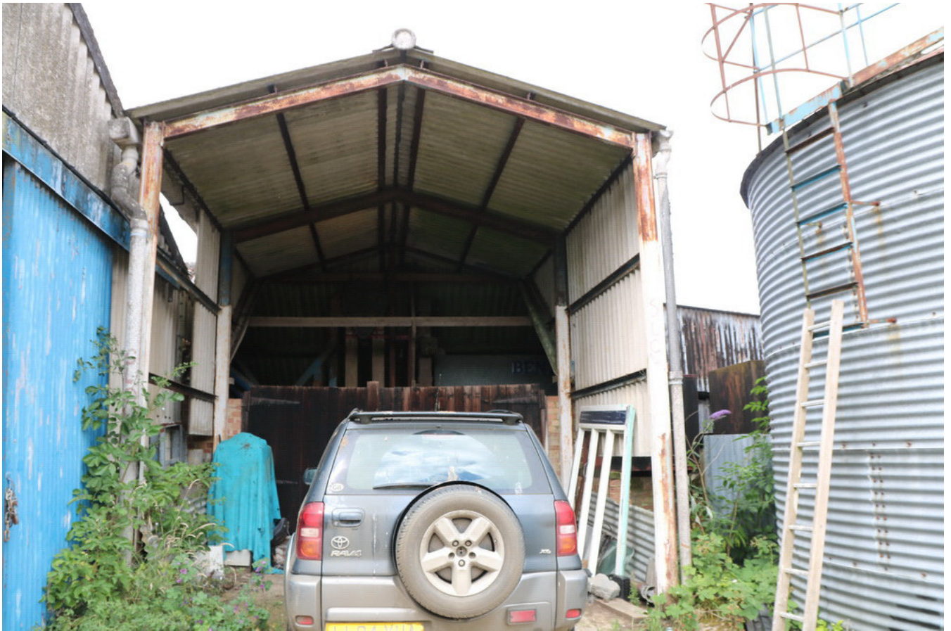
Plate 05 - Barn 2b, east elevation, facing W
