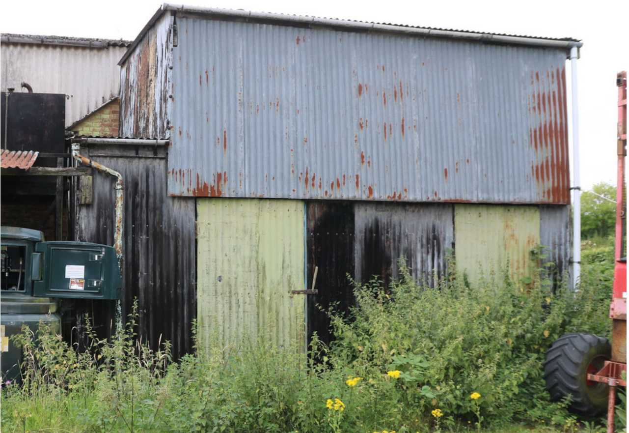
Plate 04 - Barn 2a, north elevation, facing SW
