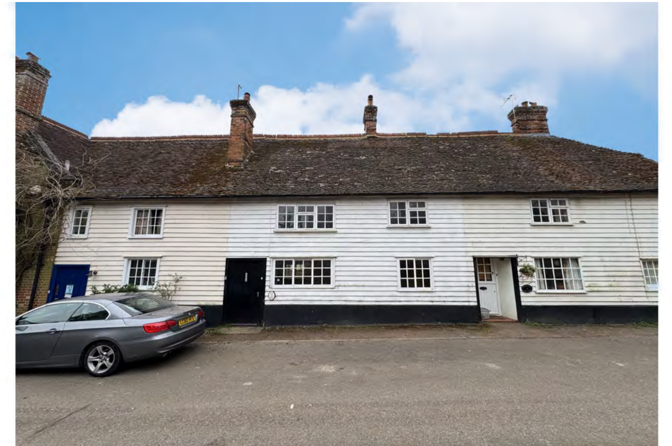
PHOTOGRAPH OF EXISTING FRONT ELEVATION
