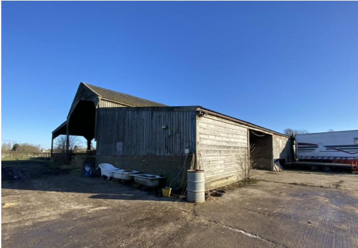
Photo 2 – Larger Stable, South and Western elevations
