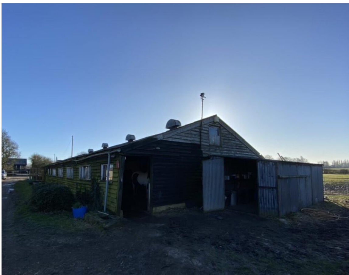
Photo 1 – Smaller Stable, West and Northern Elevations
