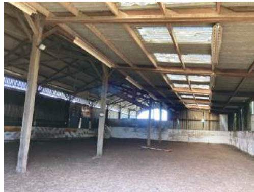
Photograph 14: Internal of B2
