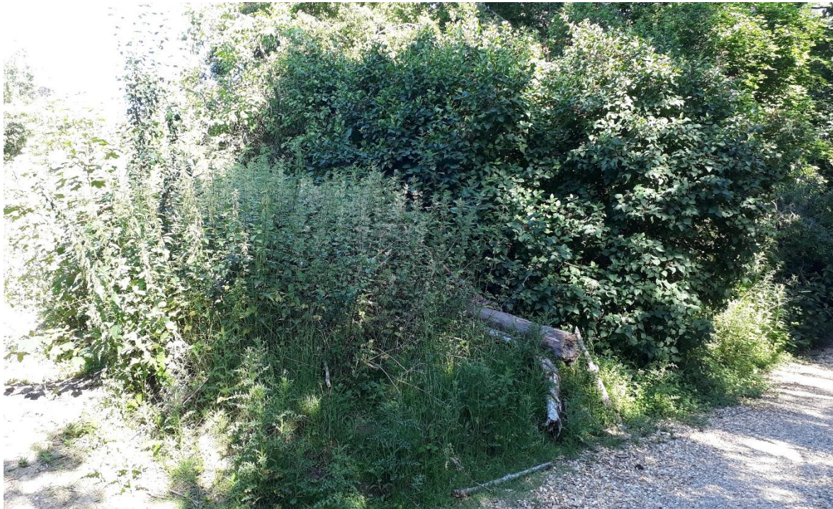
Plate 2: Overgrown embankment towards driveway.
