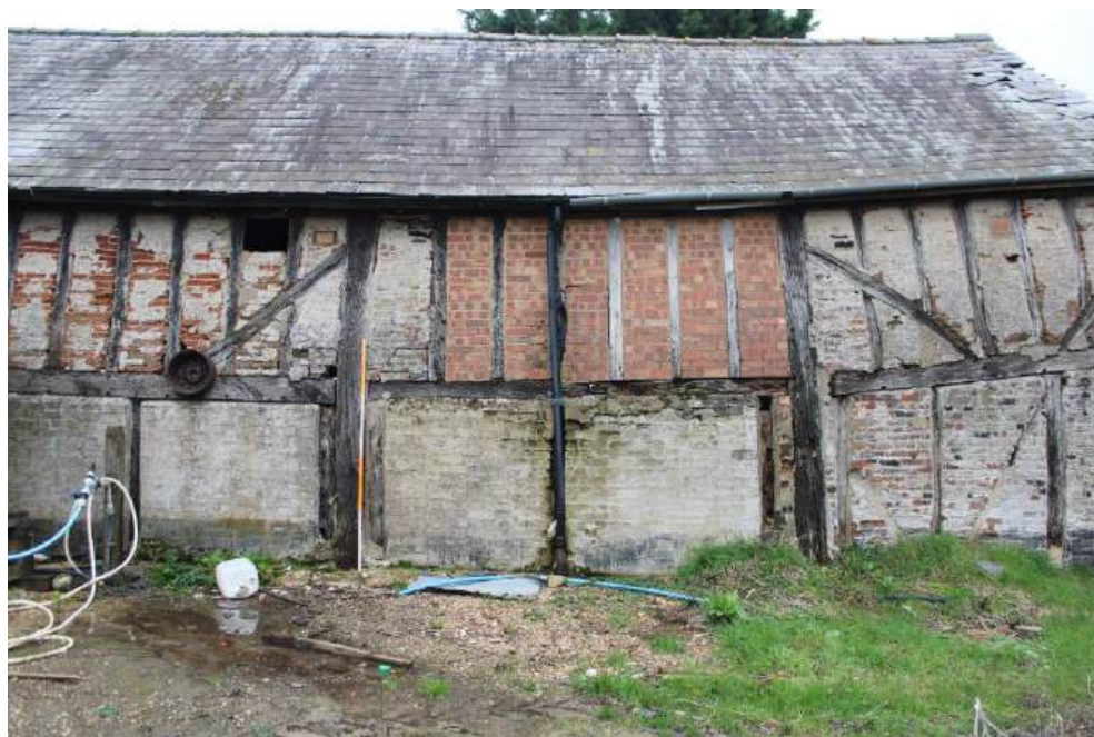
Plate 10: W-facing elevation of Barn 2 – view looking E showing timber-framed panels with close studding above and different phases of brick infill
