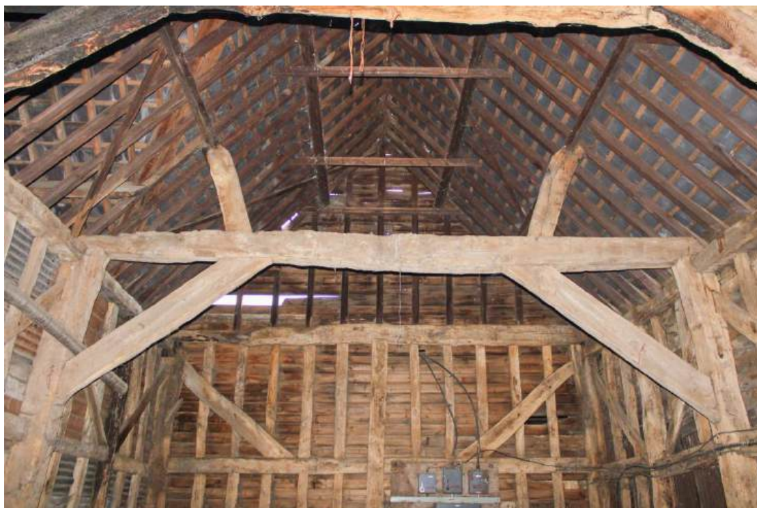
Plate 34: Internal view Barn 1 – view looking W showing detail of queen post roof truss at westernmost end of barn (Bay E)
