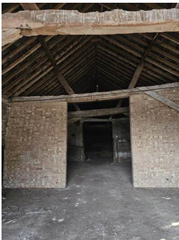
Plate 40: Internal view Barn 2 – View looking N showing detail of modern brick partition wall in central bays of barn
