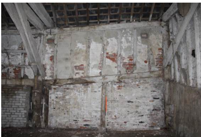
Plate 49: View looking W showing detail of timber framing in W wall of Barn 2 (Bay I)
