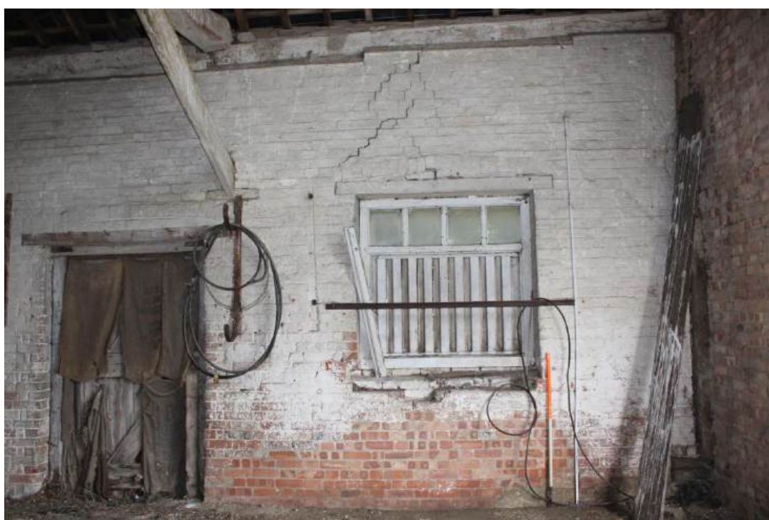
Plate 43: Internal view Barn 2 - view looking E showing detail of E wall at S end of Barn (Bay F) with window with upper glazed lights and 'hit and miss vents' and harness hook to right of doorway
