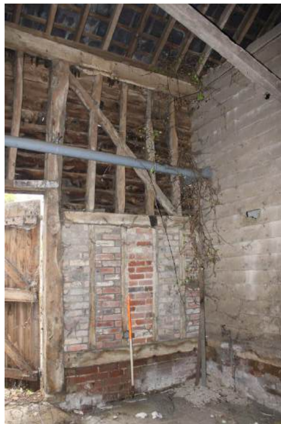
Plate 52: View looking S showing detail of partition wall with brick plinth in Barn 2 (Bay J)
