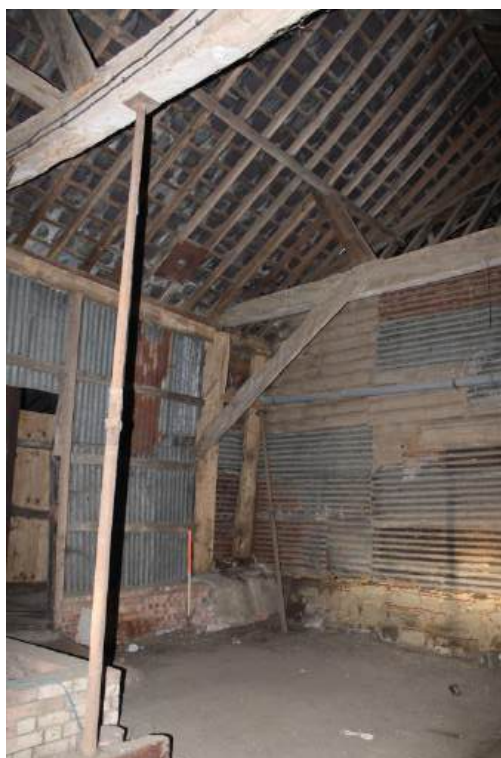
Plate 57: View looking NW showing timber framing in W wall at northernmost end of Barn 2 (Bay K)
