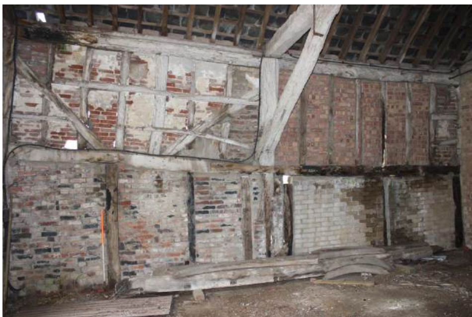
Plate 41: View looking W showing detail of timber-framed panels in southernmost bay of Barn 2 (Bay F)
