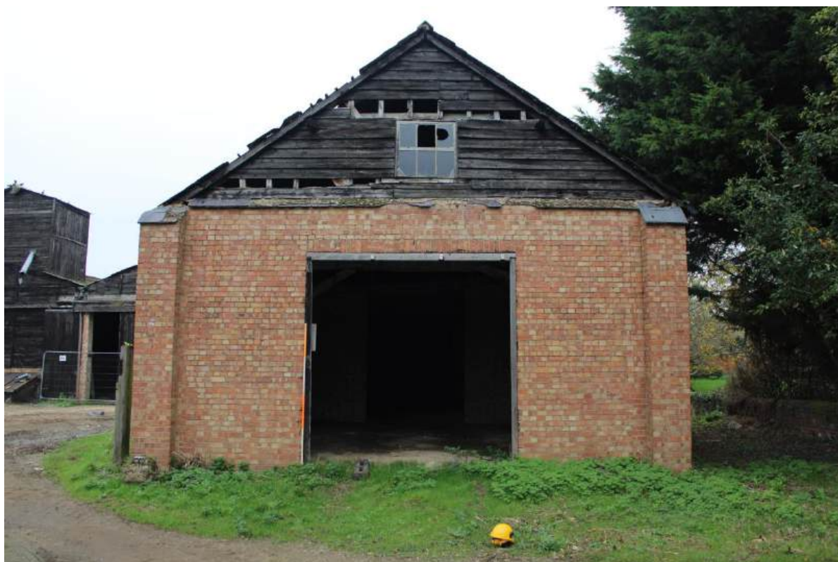
Plate 7: View N showing S gable elevation of Barn 2, reconstructed in the mid-late 20 th century
