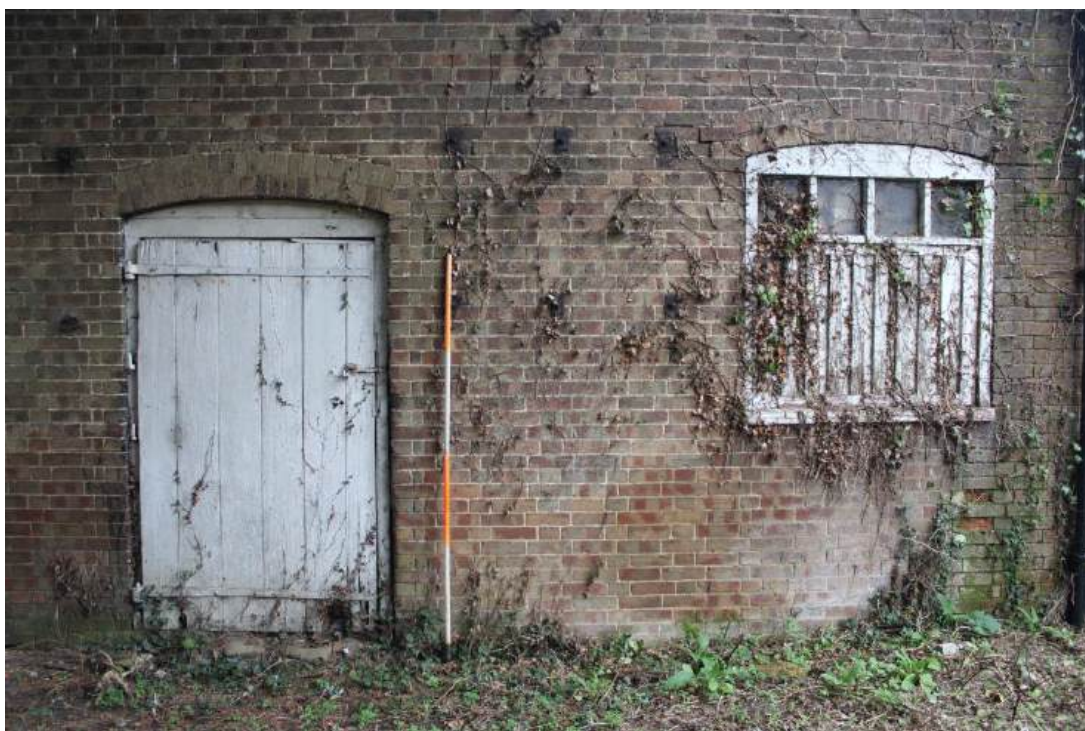
Plate 13: E-facing elevation of Barn 2 – view looking W showing detail of segmental arched doorway with plank and batten door and window with glazed upper light and wooden 'hit and miss' vents in second bay to N of the southern end of barn
