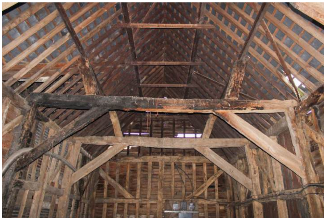
Plate 33: Internal view Barn 1 – view looking W showing detail of queen post roof truss in western portion of barn (Bay D)
