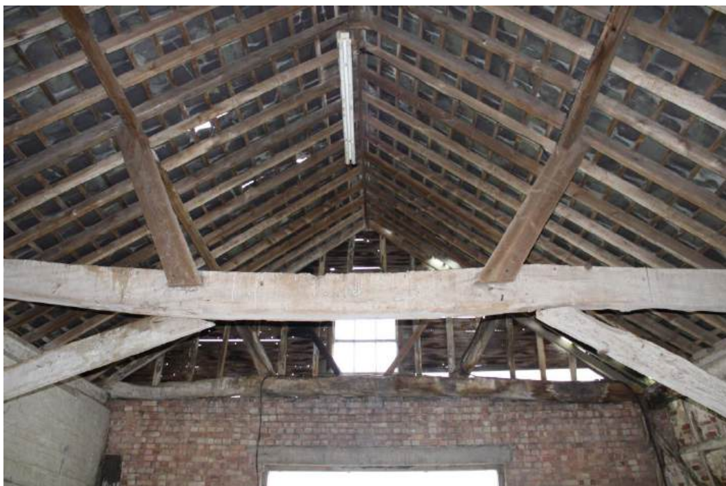
Plate 38: Internal view Barn 2 – View S towards queen post truss at S end of Barn (Bay G)
