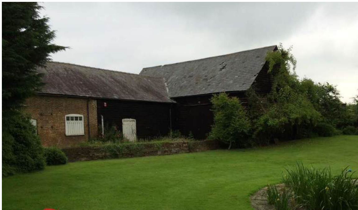
Plate 1: General view looking NW towards E gable end of Barn 1 with E elevation of Barn 2 visible to left of picture
