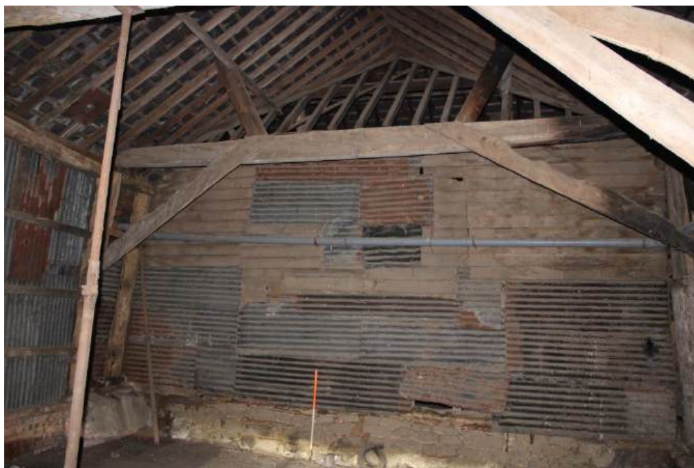
Plate 58: View looking N showing northern end of Barn 2 with queen post roof truss
