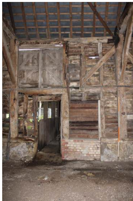
Plate 19: Internal view Barn 1 – view S showing double doors to threshing floor in Bay B
