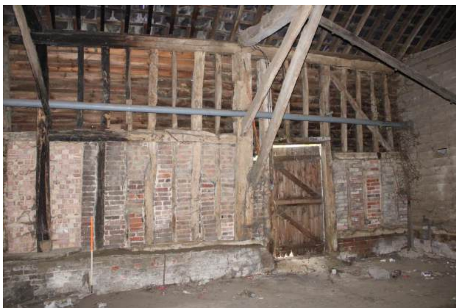
Plate 56: View looking W showing timber framing in northernmost bays of Barn 2 (Bays J & K)
