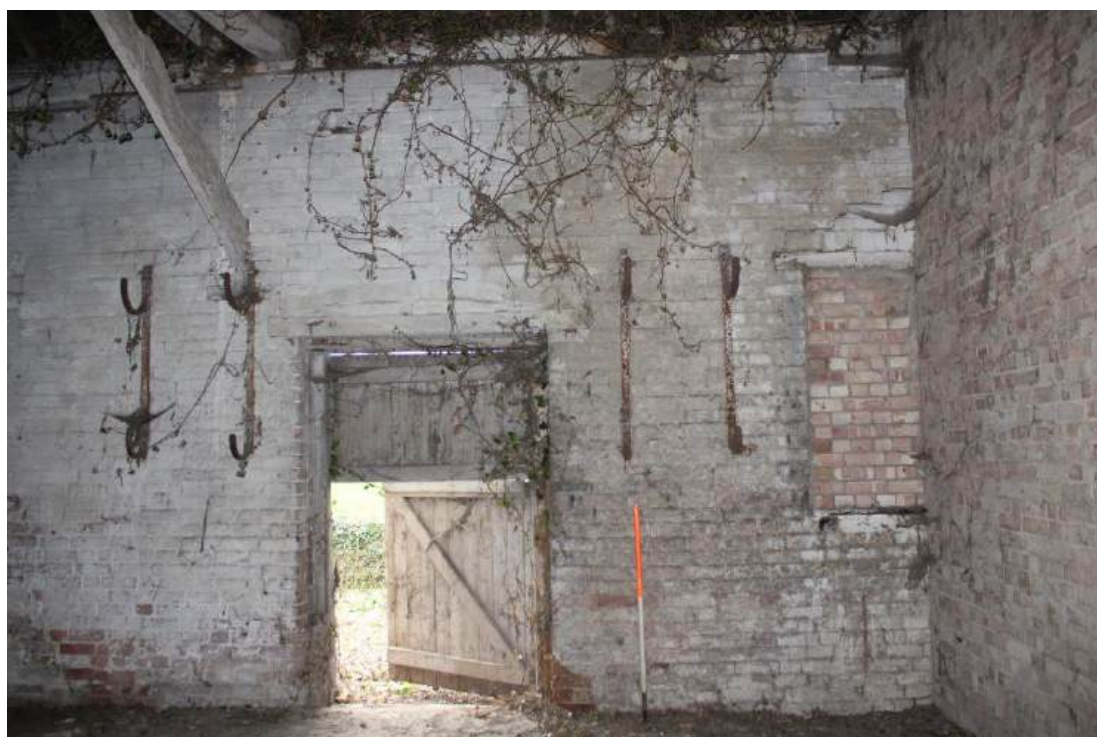
Plate 47: View looking E showing doorway flanked by harness hooks on E wall of Barn 2 (Bay H) with blocked window visible to right of picture
