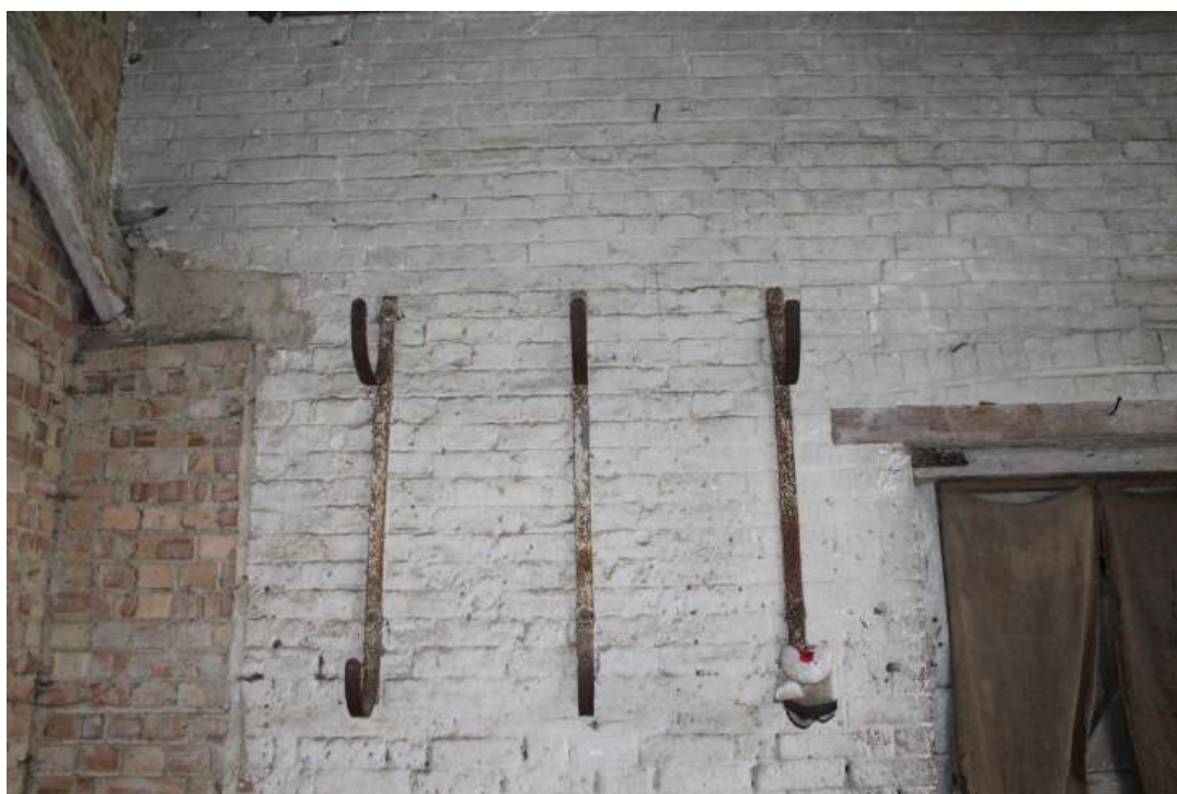
Plate 45 View looking E showing detail of wall hooks and blocked window in E wall of Barn 2 (Bay G)
