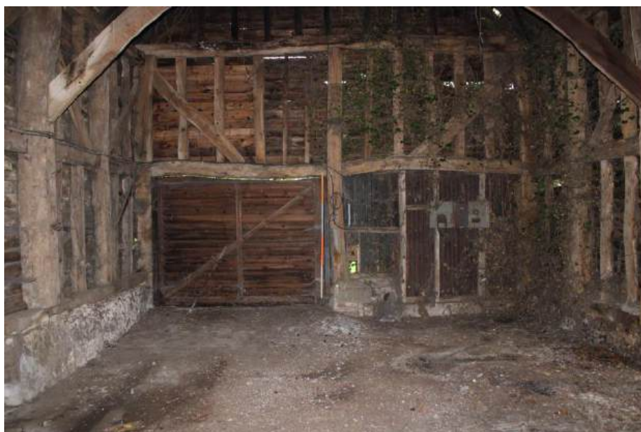
Plate 24: Internal view Barn 1 – view looking E showing eastern end of Barn 1 with modern car port door
