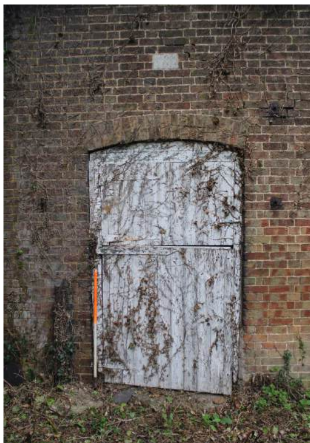
Plate 15: E-facing elevation of Barn 2 – view looking W showing detail of segmental arched doorway with double-leaf door in central bay with stone plaque above
