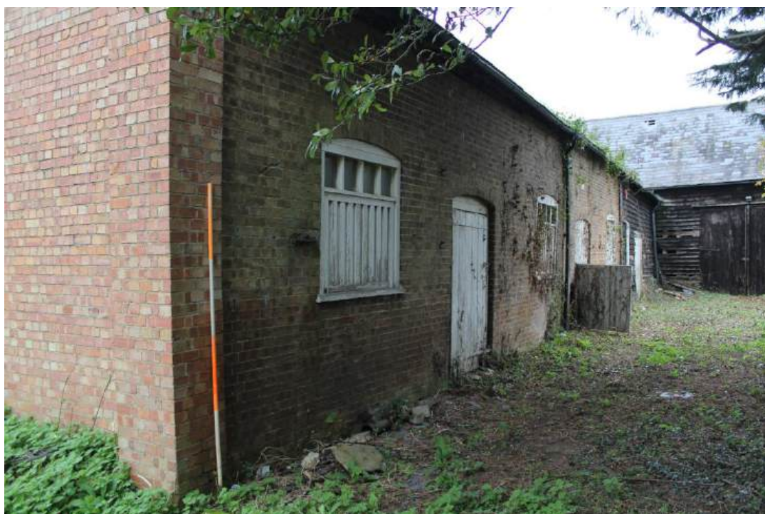
Plate 12: Oblique view NNW showing E-facing elevation of Barn 2 rebuilt in stock brick in 1873
