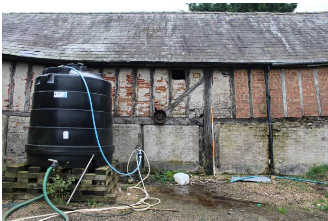
Plate 11: W-facing elevation of Barn 2 - view looking E showing detail of cast iron shaft and flywheel for engine
