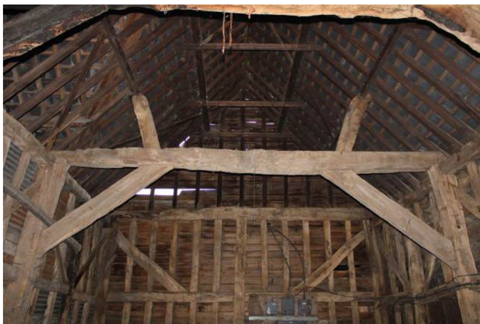
Plate 21: View looking E showing detail of Truss 1 at eastern of Barn 1
