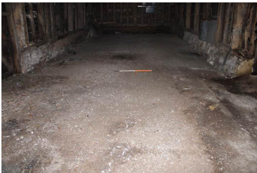
Plate 23: Internal view Barn 1 – View looking E showing detail of floor at N end of barn with possible remains of threshing floor to right of picture
