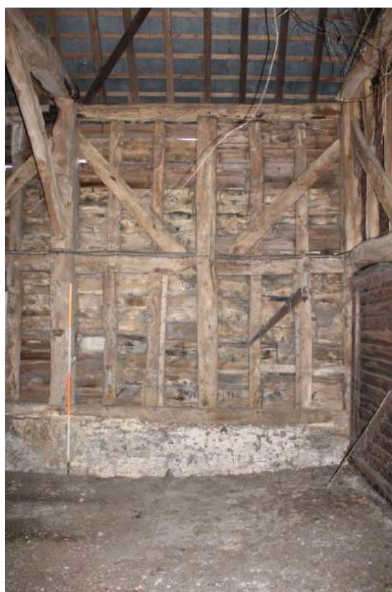
Plates 25 and 26: Internal view Barn 1 View looking N and S showing timber framing in easternmost bay of Barn
