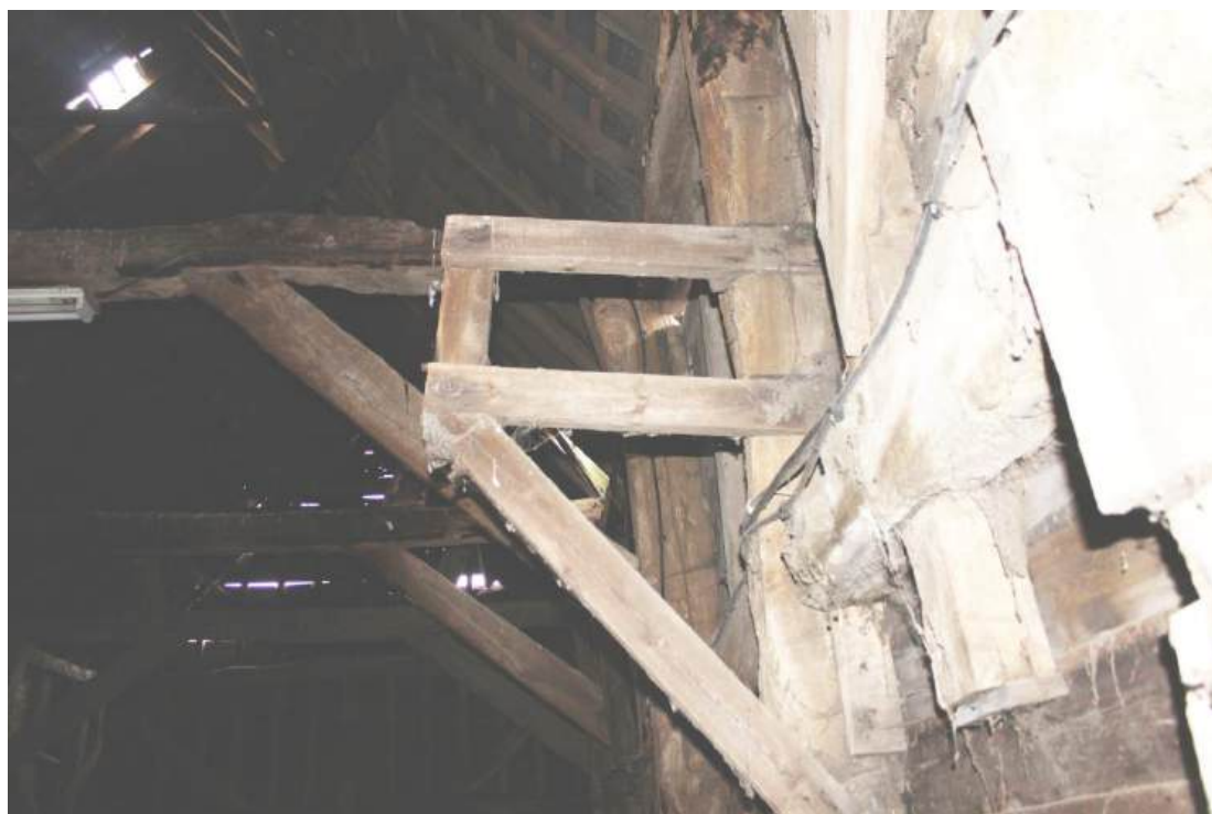
Plate 22: Internal view Barn 1 – View looking W showing detail of hoist above doorway in N wall
