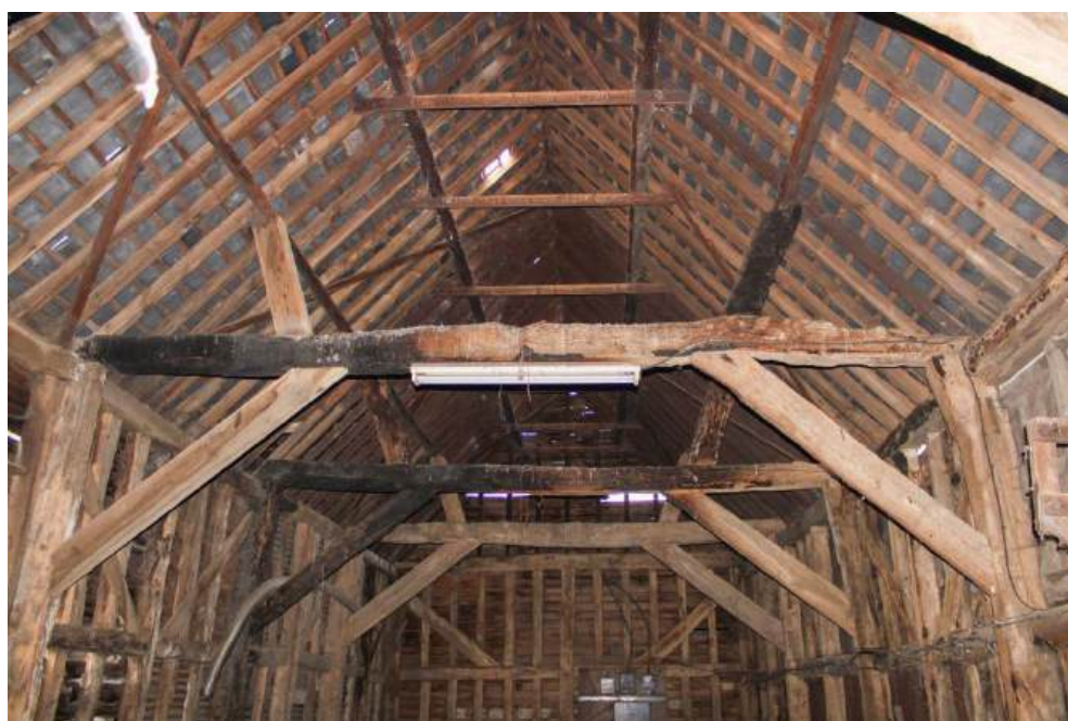
Plate 28: Internal view Barn 1 – view looking W showing queenpost roof trusses in central and western bays
