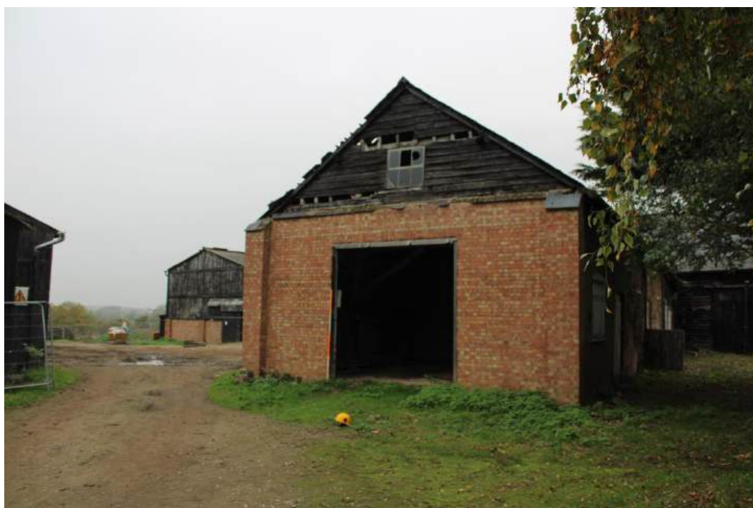
Plate 6: General view looking NNW showing S gable end of Barn 2, reconstructed in modern brick with late 20 th century barns visible in background to left of picture
