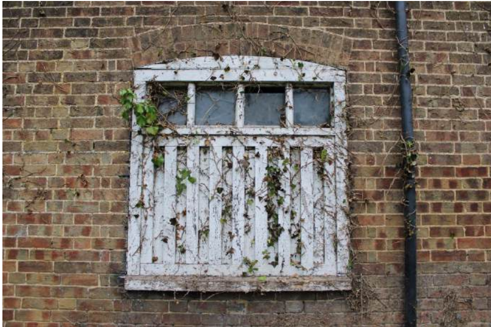
Plate 17: E-facing elevation of Barn 2 – view looking W showing detail of window to right of central doorway with glazed upper lights and 'hit and miss' vents
