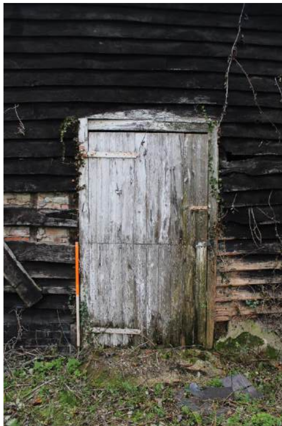
Plate 18: E-facing elevation – View W showing detail of doorway in northernmost section of Barn 2
