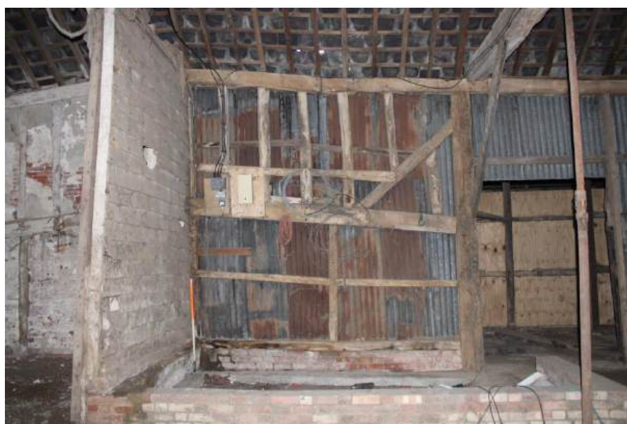
Plate 54: View looking W in Barn 2 showing detail of brick engine base at N end of barn (Bay J) with timber framing of W wall in background and doorway to modern barns to right of picture
