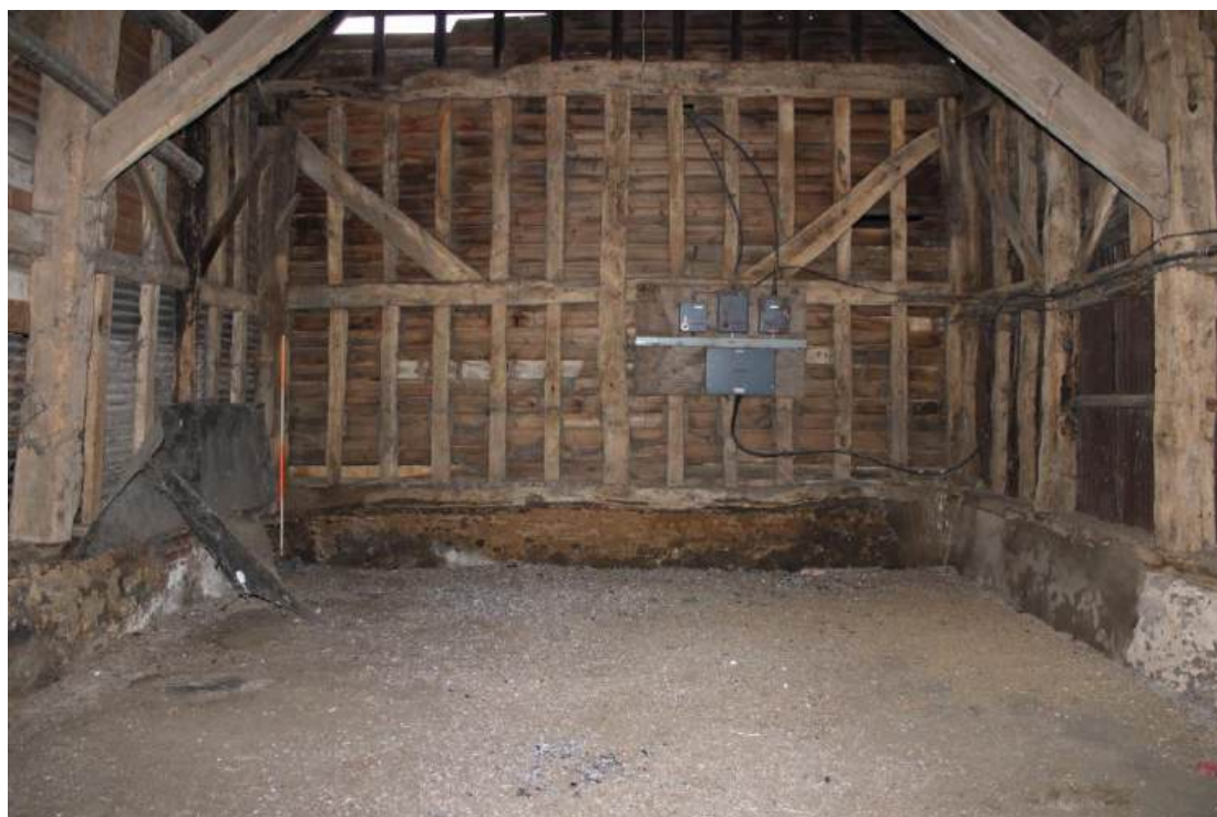
Plate 35: Internal view Barn 1 – view looking W showing close studded timber-framing at W end of barn
