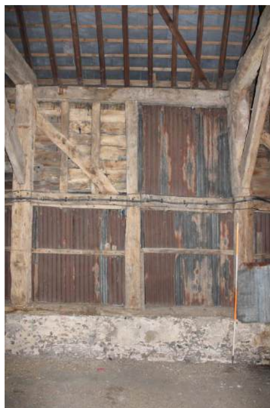
Plates 31 & 32 : Internal View barn 1 - View looking N and S showing detail of timber framing in Bay D
