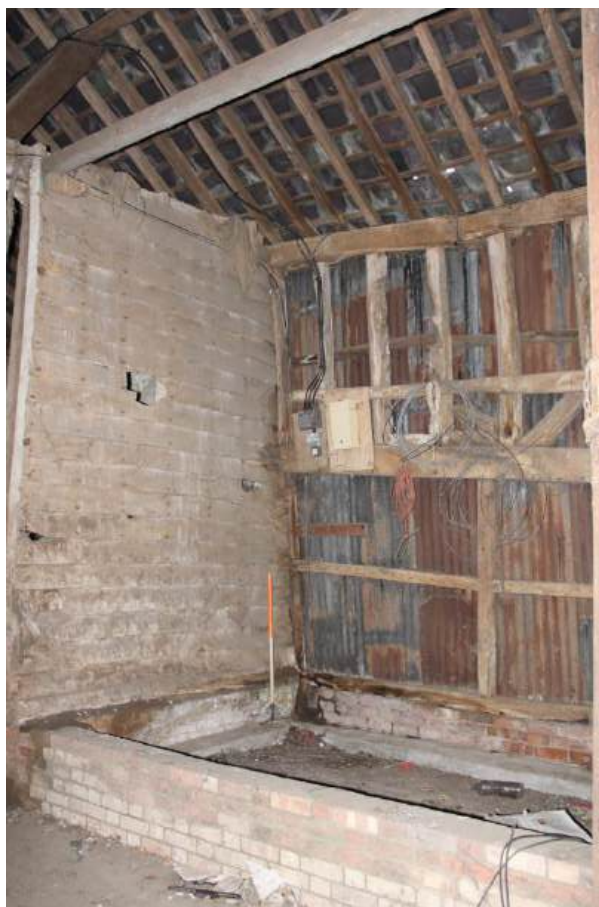
Plate 55: View looking SW showing detail of engine base and partition wall in Barn 2 (Bay J)
