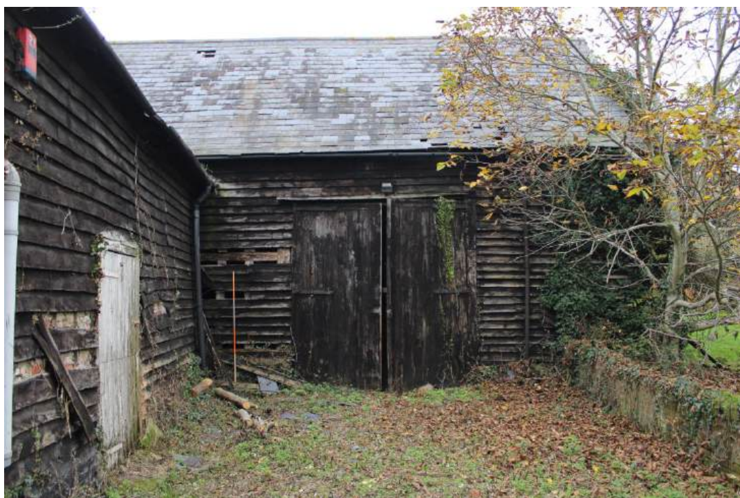
Plate 2: View looking N towards eastern end of S-facing elevation of Barn 1, showing double doors
