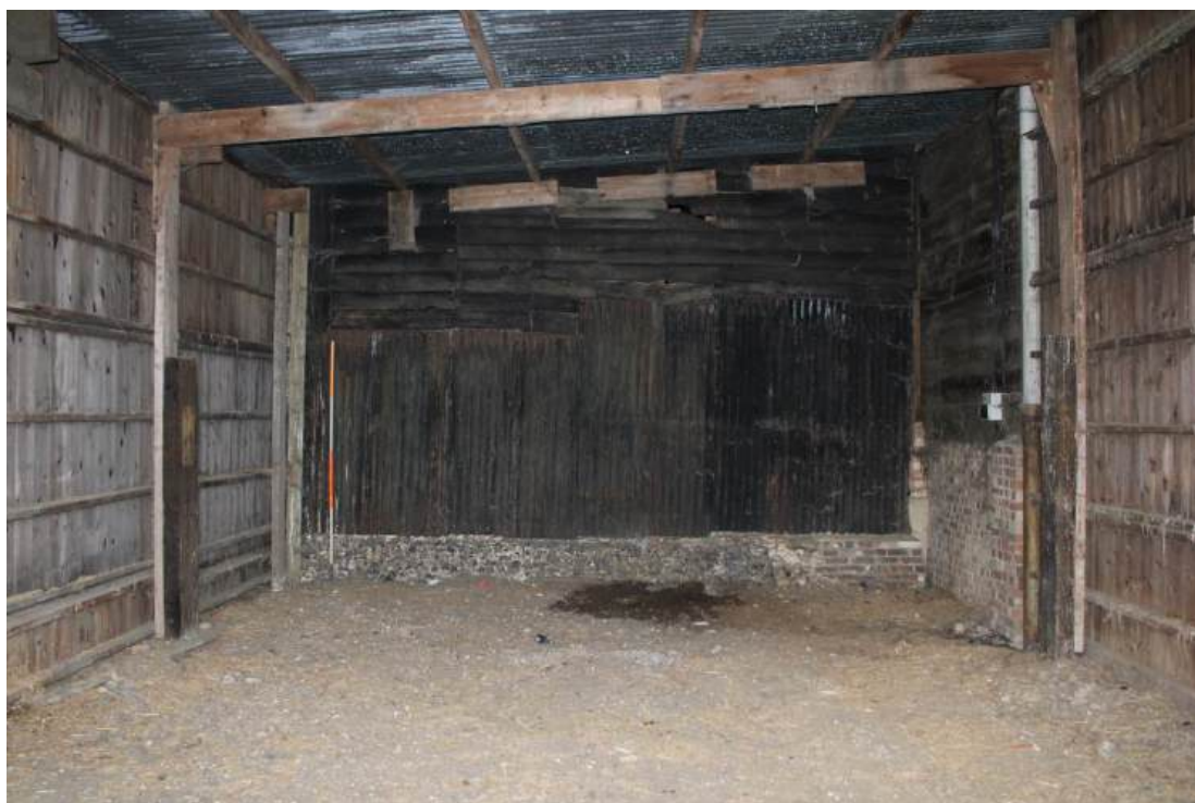
Plate 5: View looking S from open fronted shed showing W end of N-facing elevation of Barn 1 with stone plinth visible beneath weatherboarding and corrugated metal cladding
