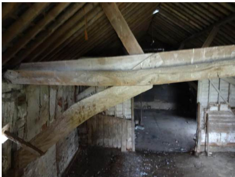
Plate 46: Internal view Barn 2 – view looking N showing detail of queen post roof truss with curved struts between bays H and I
