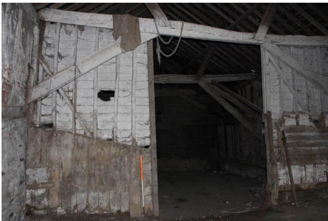
Plate 51: View looking N showing partition wall with brick plinth in Barn 2 (Bay I)
