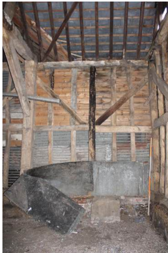
Plates 36 & 37 Internal view Barn 1 – views looking N and S showing detail of timber framing in westernmost bay (Bay E)
