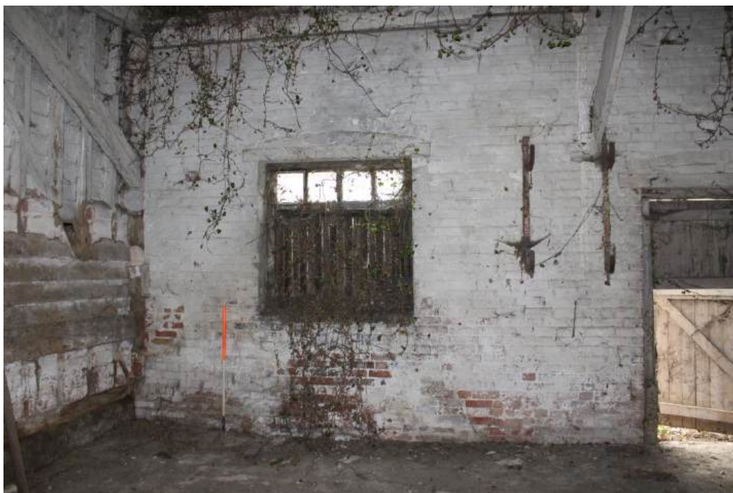
Plate 50: View looking E showing detail of window in E wall of Barn 2 with doorway to right (Bay I)
