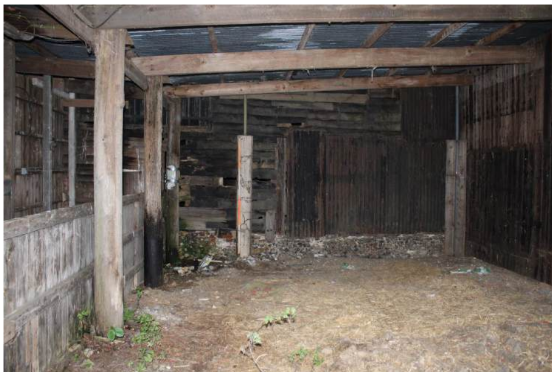
Plate 4: View looking S showing central portion of N-facing elevation of Barn 1 with timber framed structure resting on stone masonry plinth and weatherboard cladding partially replaced by modern corrugated metal sheeting
