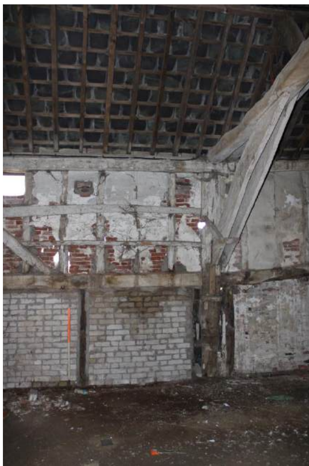
Plate 48: View looking W showing detail of timber framing in W elevation of Barn 2 (Bay H)
