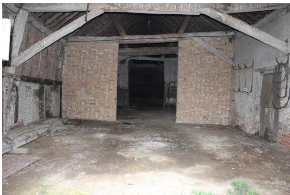
Plate 39: Internal view Barn 2 – view looking N showing interior of S part of barn with modern brick partition
