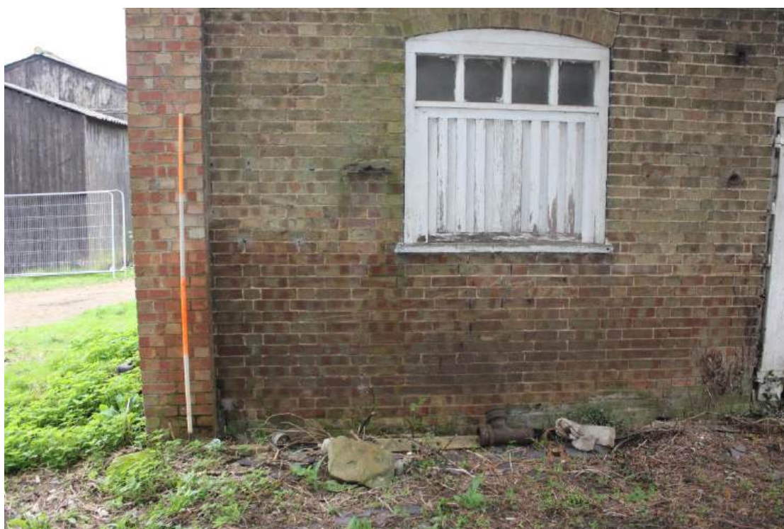
Plate 14: E-facing elevation of Barn 2 - view looking W showing detail of segmental arched window with glazed upper light and wooden 'hit and miss' vents to left of doorway at southern end of barn
