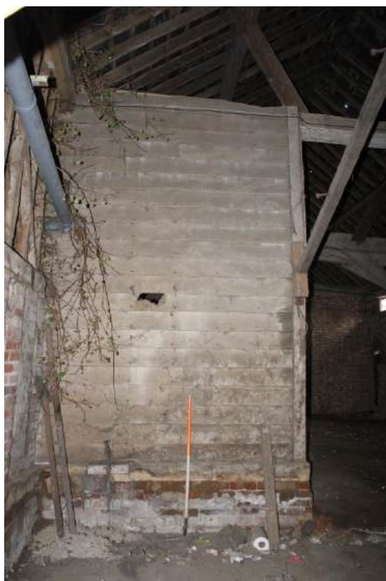
Plate 52: View looking S showing detail of partition wall with brick plinth in Barn 2 (Bay J)
