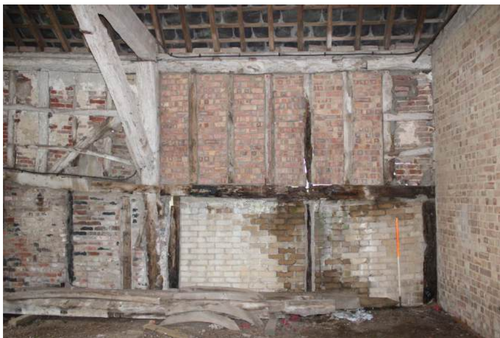
Plate 42: View looking W showing detail of timber framed panels with modern brick infill in W elevation of Barn 2 (Bay G)
