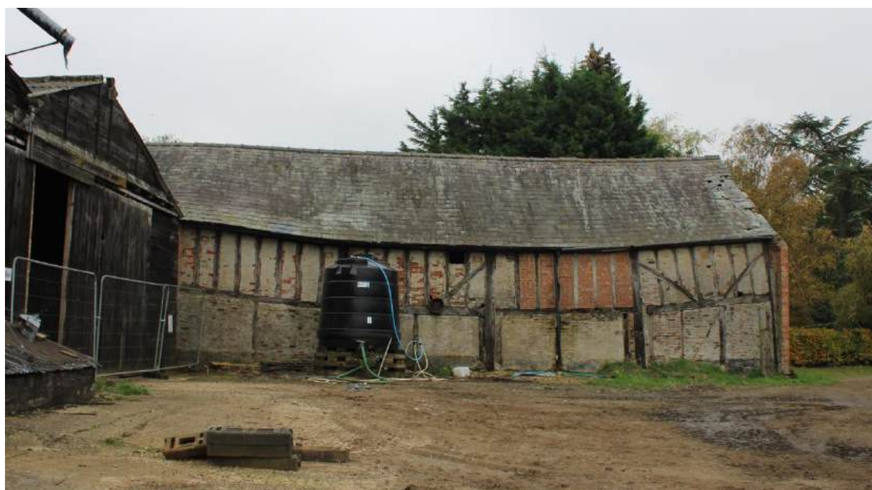
Plate 8: General view looking E showing W-facing elevation of Barn 2
