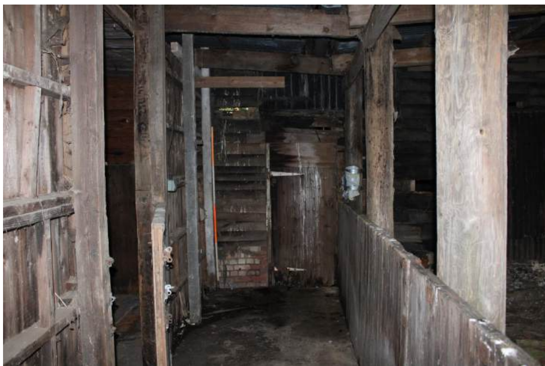
Plate 3: View looking S from open fronted shed showing 'winnowing door' in N-facing elevation of Barn 1 with loading bay hatch above
