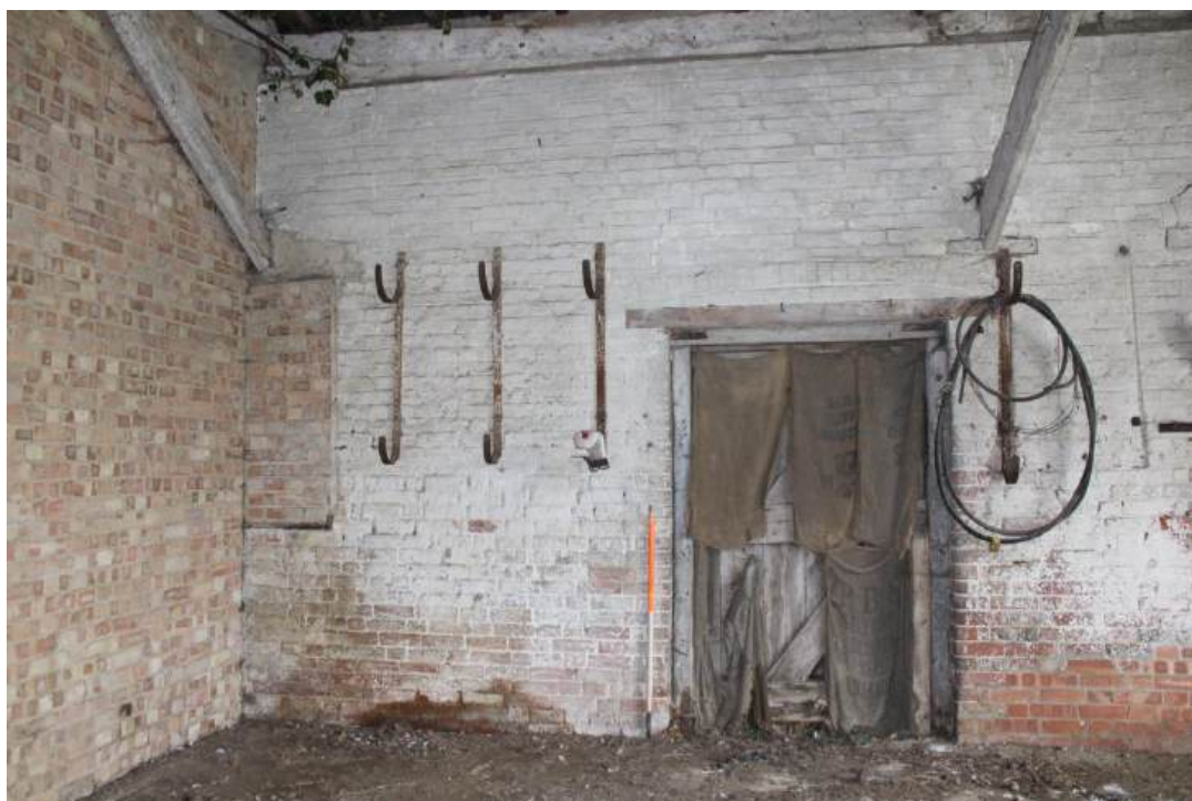
Plate 44: Internal view Barn 2 – view looking E showing door in E wall with flanking harness hooks and blocked window to left, blocked as a result of the construction of the modern brick partition wall
