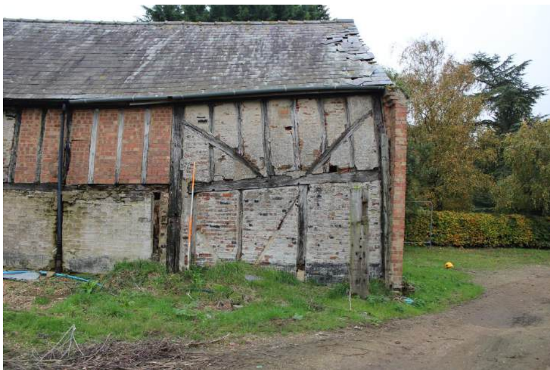
Plate 9: W-facing elevation of Barn 2 – view looking E showing detail of timber-framing with brick nogging in southernmost bays
