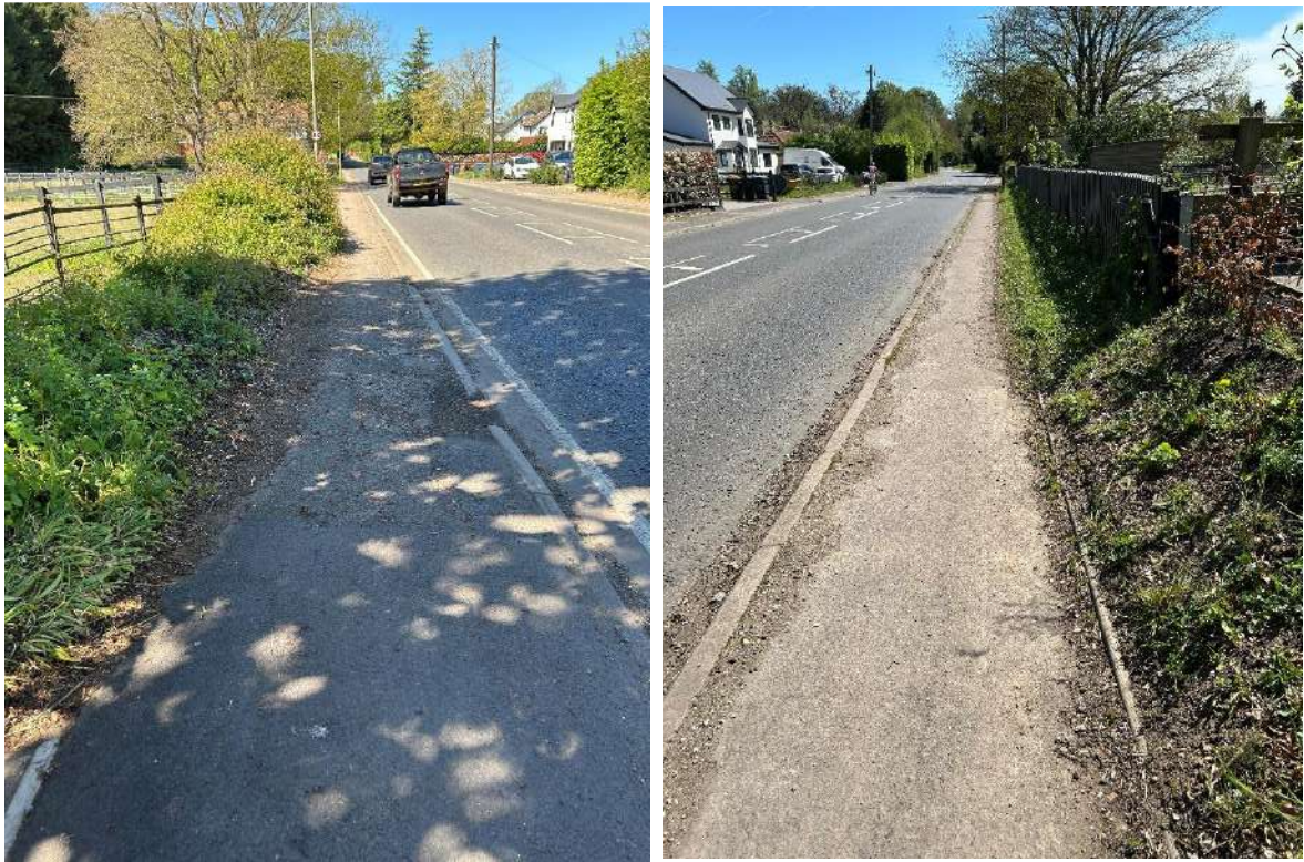
Existing footway to be cleared along the site frontage
