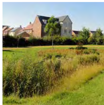
Sustainable drainage ponds and swales capture and hold excessive rainfall
