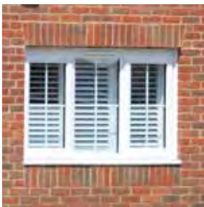
Brick window headers & cills
