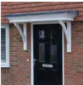
Flat roof porch
