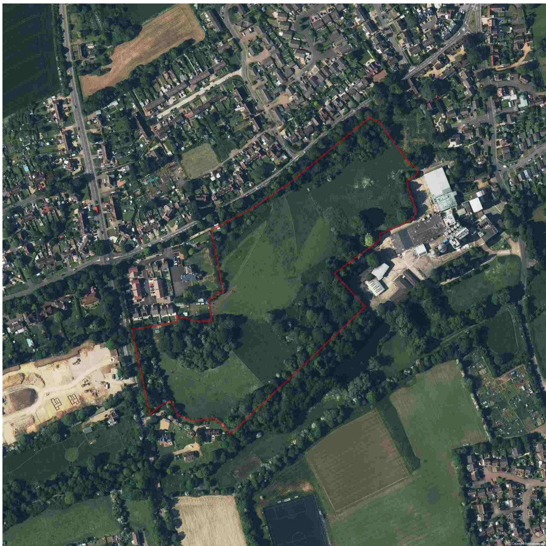
Figure 1: Site location. Land at Ickleford Manor, Turnpike Lane, Ickleford, Hertfordshire, SG5 3XD. Photograph capture Date: 27 th May 2023. (Reproduced with permission from Groundsure.) The red line does not imply ownership or a development boundary.
