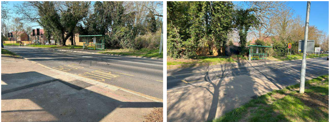
Figure 4 Bedford Road – Bus Stops
