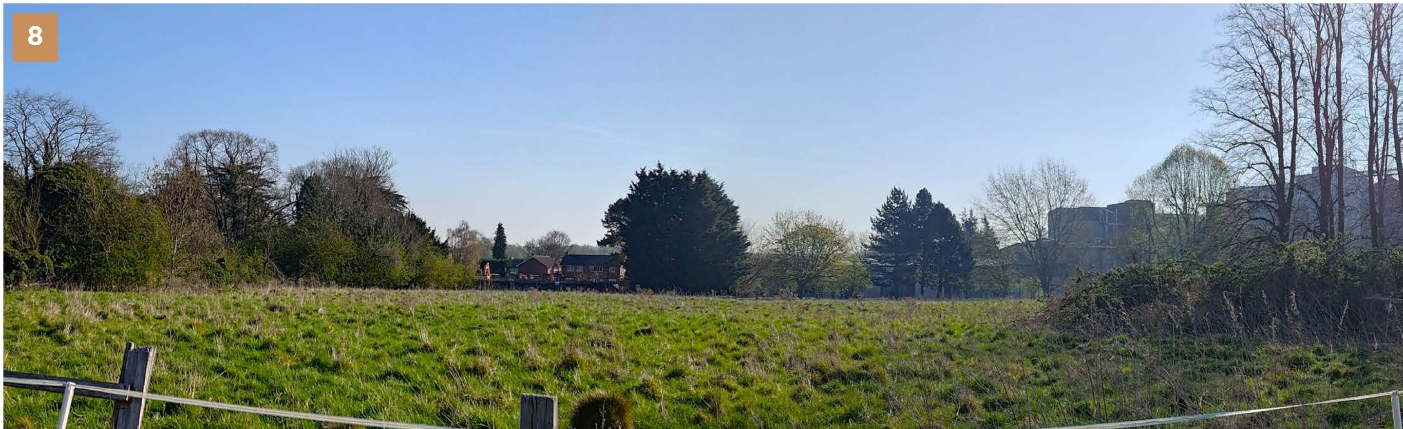
VIEW SOUTHEAST TOWARD DISUSED FLOUR MILL
