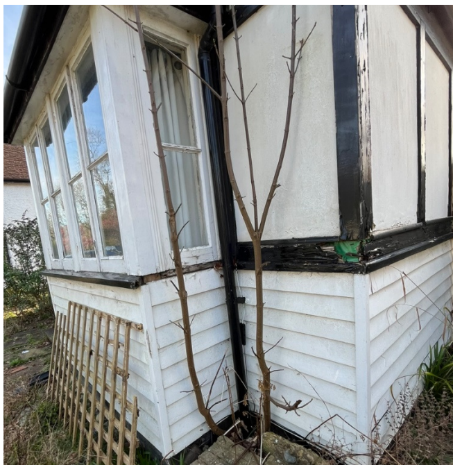
Exposed existing timber frame
