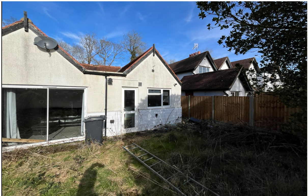
Rear elevation viewing 213 Icknield Lane
