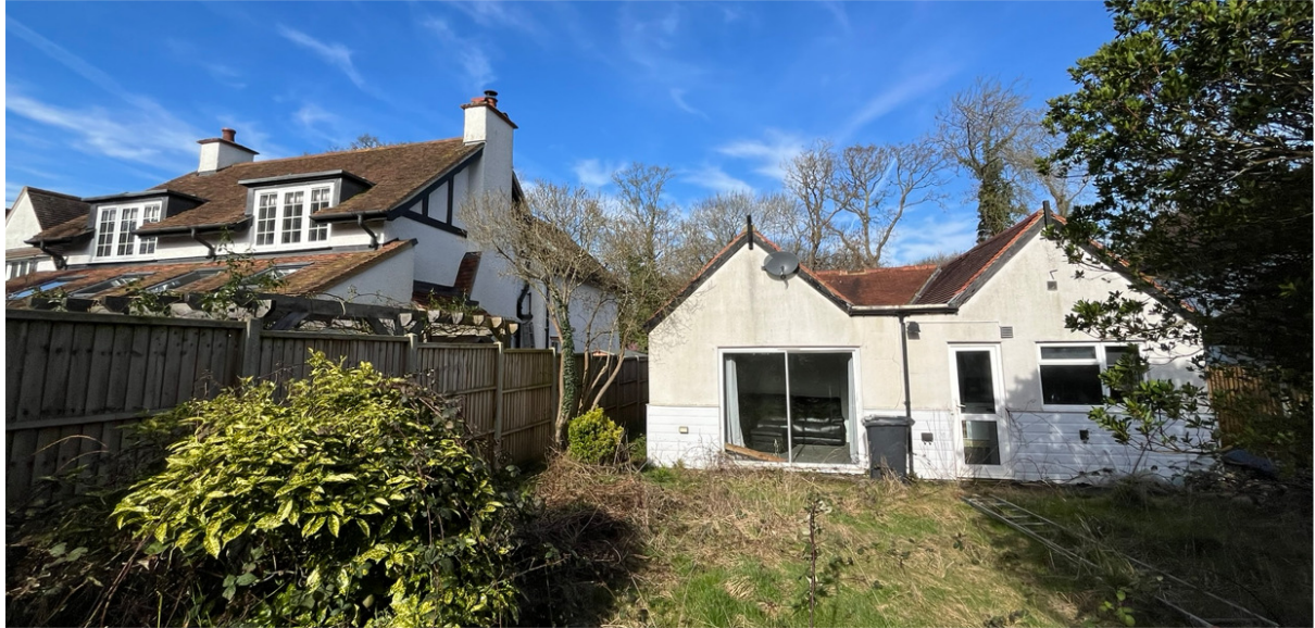
Rear elevation viewing 209 Icknield Lane
