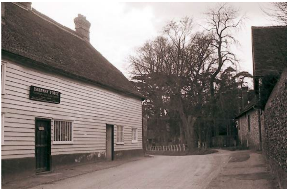
Fig 4 – Old archive picture showing the forge and no street facing front windows at first floor
