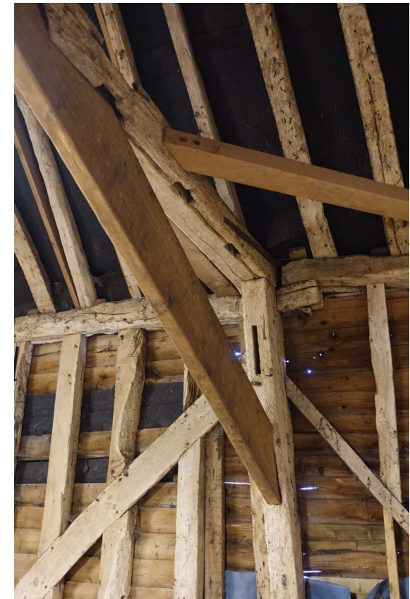
Fig. 8 ( above ): The post and truss at the south end of Bay 5, formerly the end (west) wall of the barn; note the mortices for downward braces and studs, and the lighter studwork in Bay 6 (right-hand side of photo).
