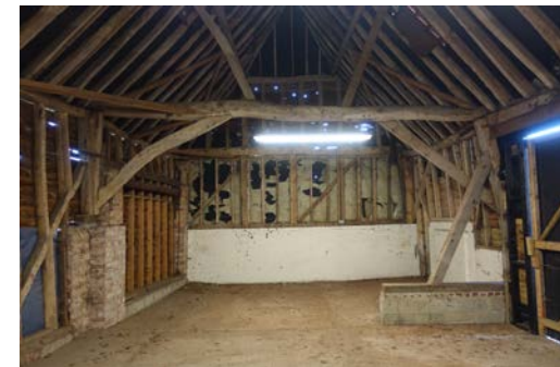
Fig. 11: Bays 6 and 7 looking west – later and more altered than bays 1 to 5.
