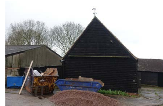
Fig. 14: East end of the barn; note the lean to the left (south).
