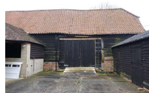
Fig. 12: The much-altered western cart entrance on the north side of the barn (Bay 6).
