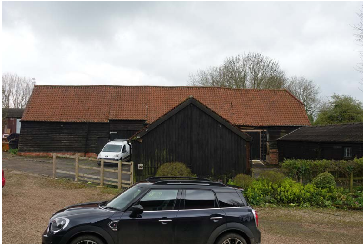
Fig. 4: View south from the farmhouse to the barn, with the shelter shed in front and stables to the right.
