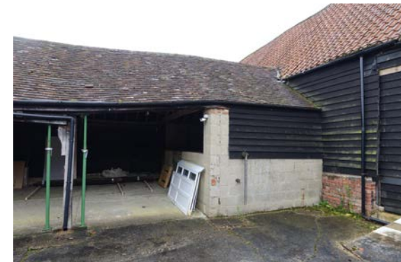
Fig. 21: The junction between the shelter shed and barn.
