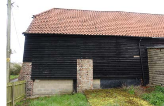
Fig. 13: west end of the south wall, showing the blocked opening between brick piers, overlaid with weatherboarding.
