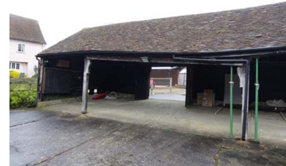
Fig. 20: View of the open (west) side of the shelter shed.
