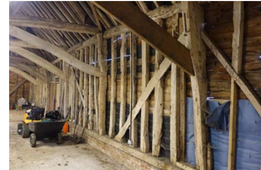
Fig. 10: The south wall of bays 1 to 5 (and part of Bay 6), showing a mixture of old and new timbers.
