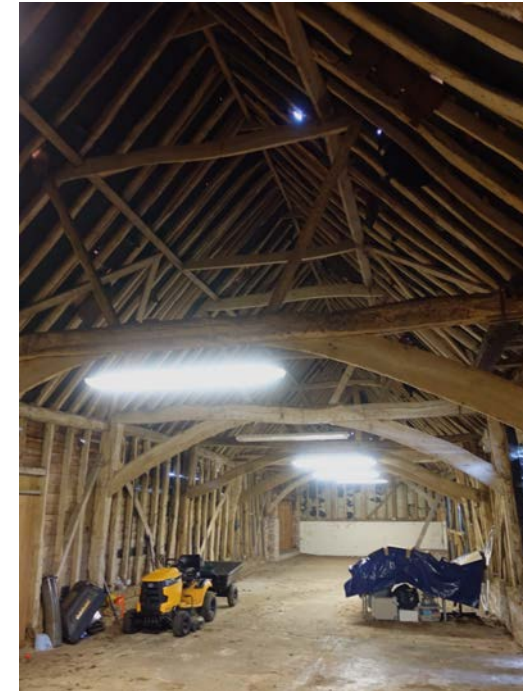
Fig. 16: General view of the interior looking west.
