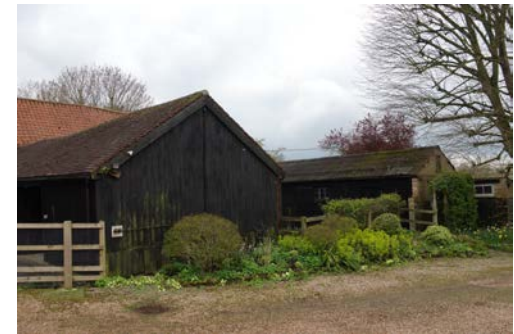
Fig. 6: The shelter shed and stables, with the roof of the barn glimpsed behind them.
