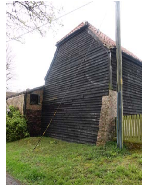
Fig. 15: West end of the barn.
