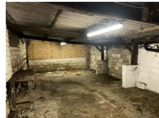
Fig. 17: Interior of the lean-to addition.
