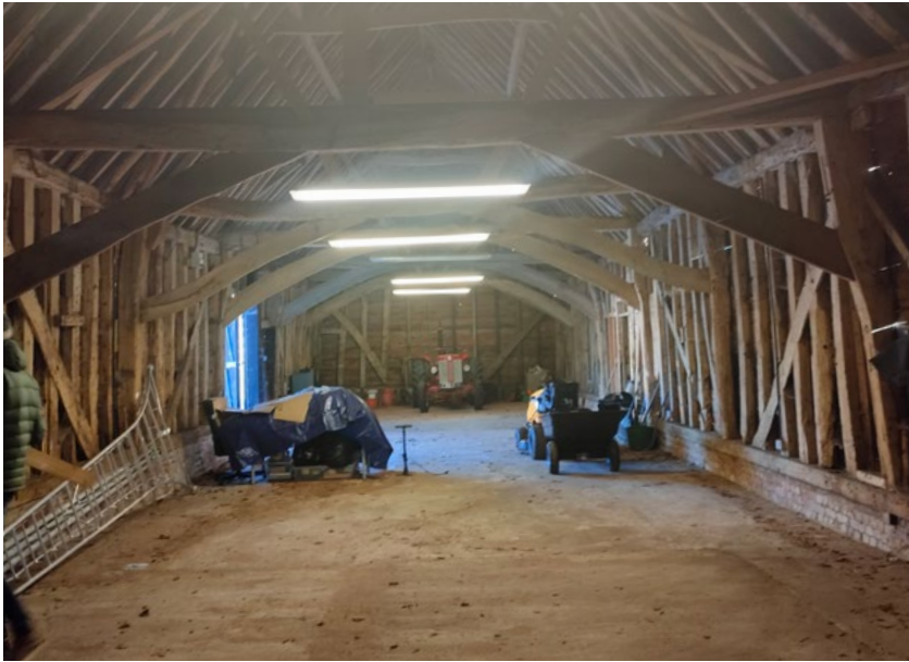
Figure Desc. The Barn, Internal View Showing Roof Trusses and the 7 Bays - Direction East
