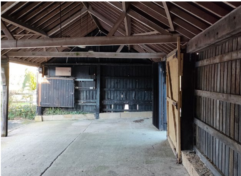
Car port structure, view facing north west
