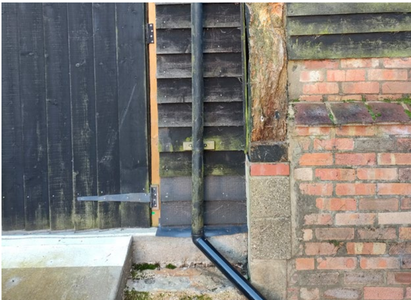
Figure Desc. Original Barn Entrance Door and RWP
