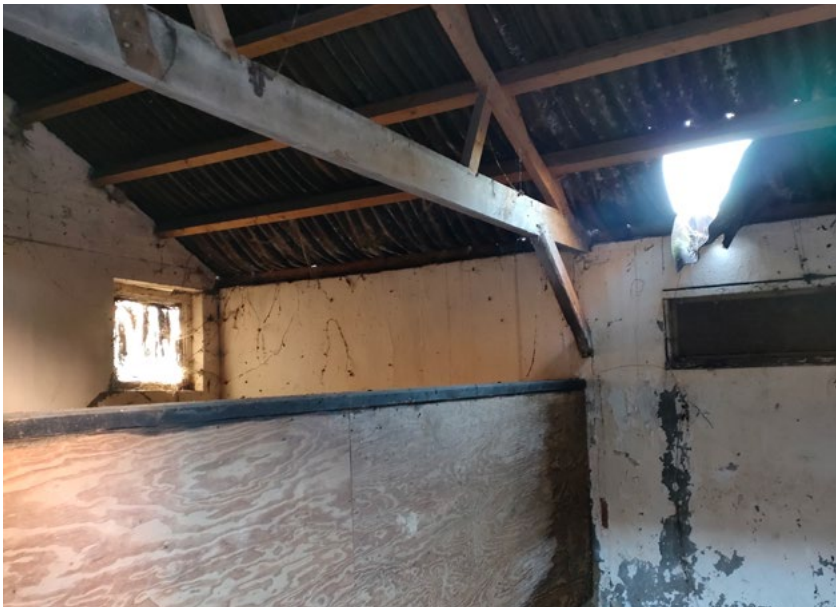
Stables building, gable end facing south eastwards
