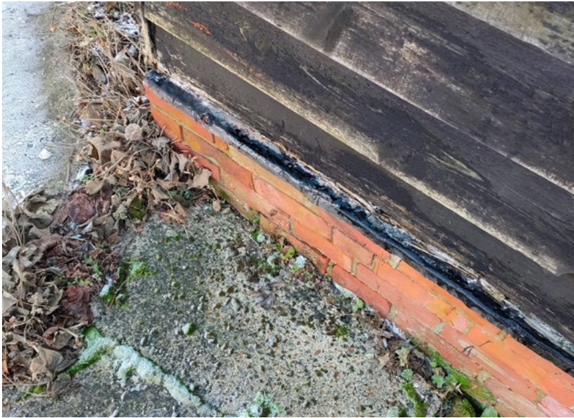
Installed DPC to underside of timber sole plate
