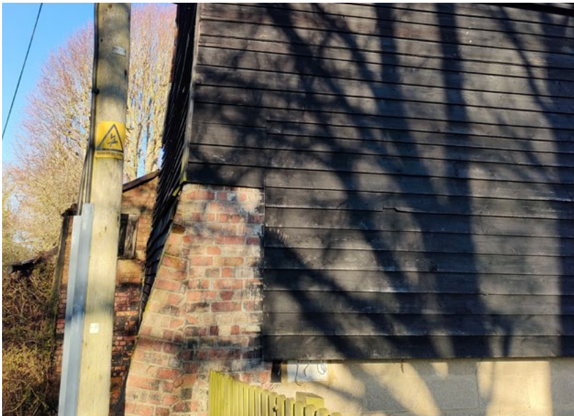
Figure Desc. The Barn, Buttreassing to corner - Direction South East
