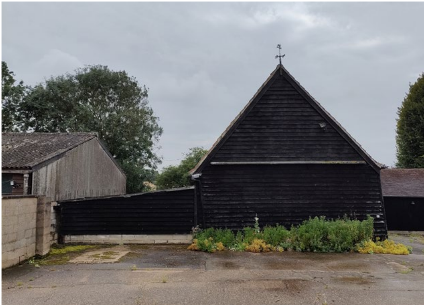
Figure Desc. (3) Grade II Listed Agricultural Barn, North Elevation
