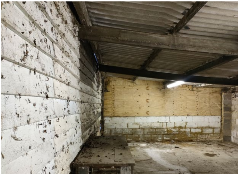
Lean-to extension, view facing north east
