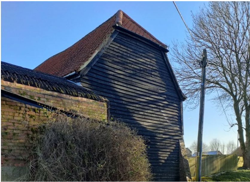
Figure Desc. The Barn, Hipped Gable End Elevation Facing Dane End Road - Direction South East
