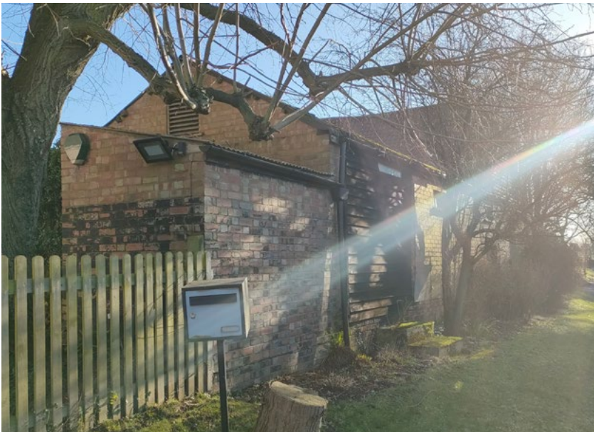
Figure Desc. 19th C Extension, Facade Facing Dane End Road - Direction South East
