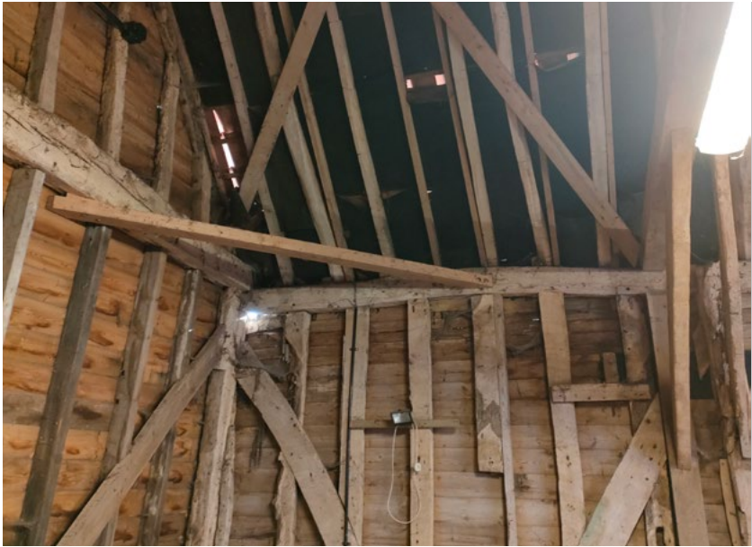
Introduction of new timber framing to provide additional stability to existing timber frame
