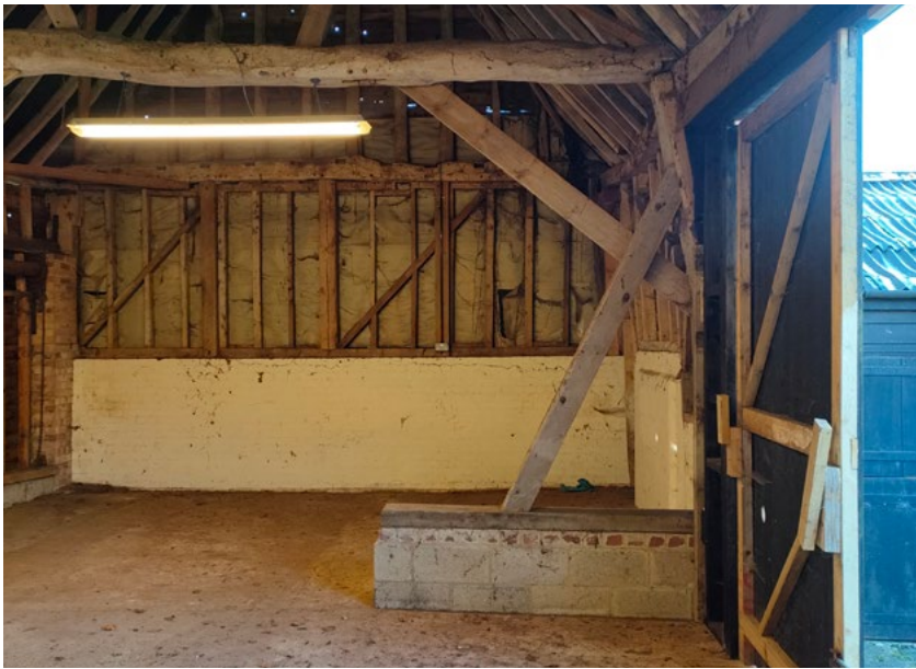
Blockwork dwarf walling and support existing timber frame structure
