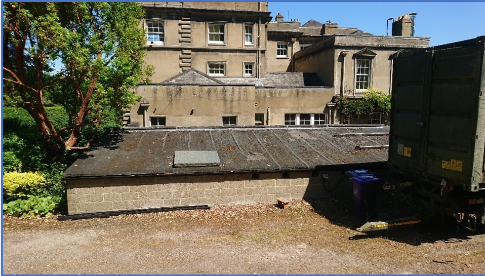
Figure 3 – View of service building rear elevation, from adjacent higher ground level
