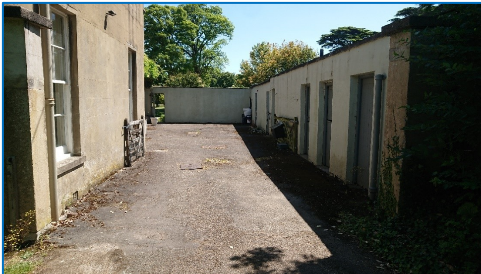
Figure 2 – View of the service outbuilding alongside Hexton Manor
