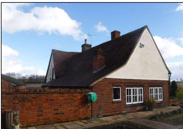
Figure 9. Walnut Tree Farmhouse, viewed from the west – gable end of rear wing
