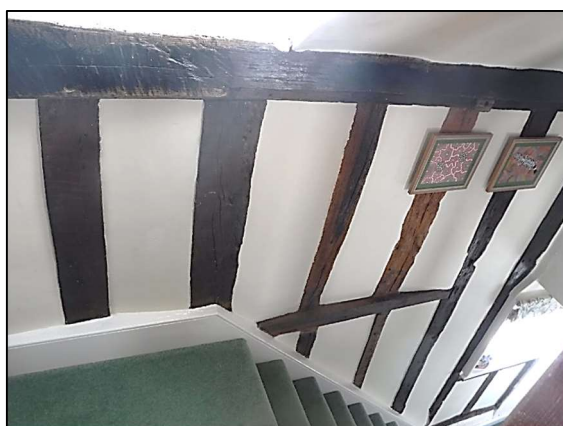
Figure 12. Timber frame to rear wall of front range
