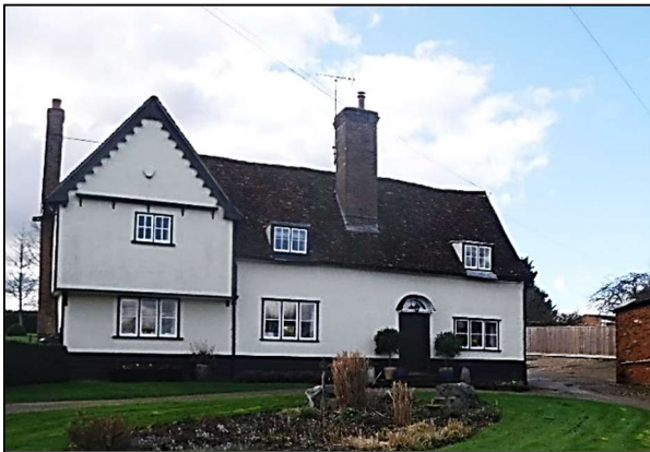
Figure 7. Walnut Tree Farmhouse, east (front) elevation
