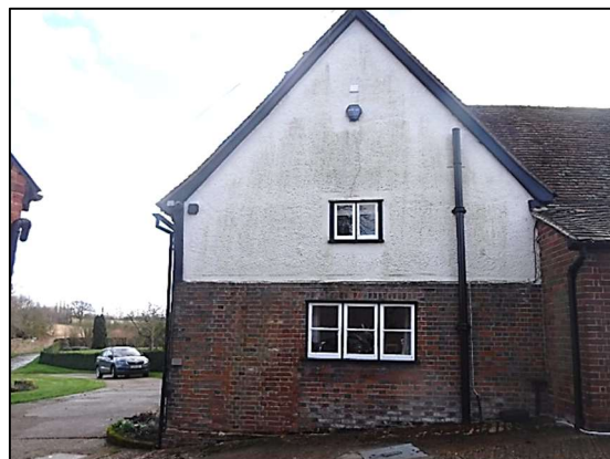
Figure 10. Walnut Tree Farmhouse, north gable end of front / east range
