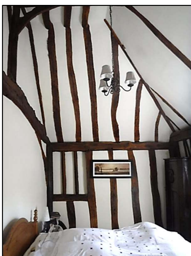
Figure 11. Timber frame to cross wing, first floor
