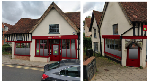
Building once work carried out
