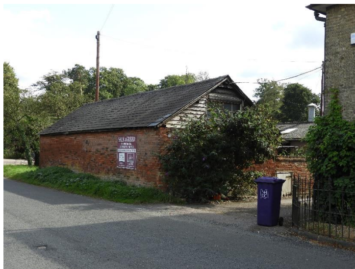
C19th brick barn on application site frontage.
