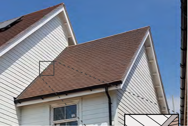
Maintain a min. 50 mm clearance between Hardie® VL Plank weatherboard and a hard surface eg. roofs and concrete paths, steps and driveways.
