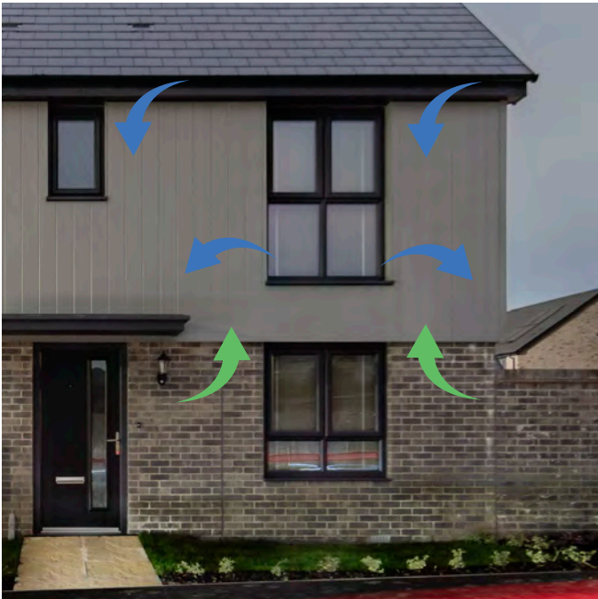
→ Green: Air inlets → Blue: Air Outlets
