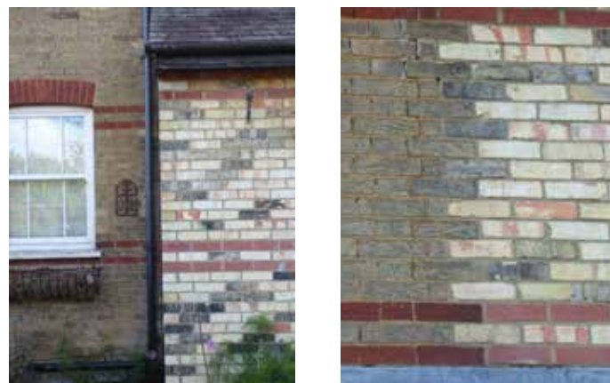
Figure 106: Poorly matched, bright modern brick, can contrast poorly next to original buildings if not well considered
