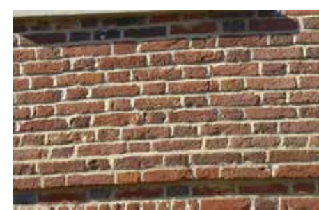
Figure 43: Example of Flemish bond brickwork with imperial bricks
