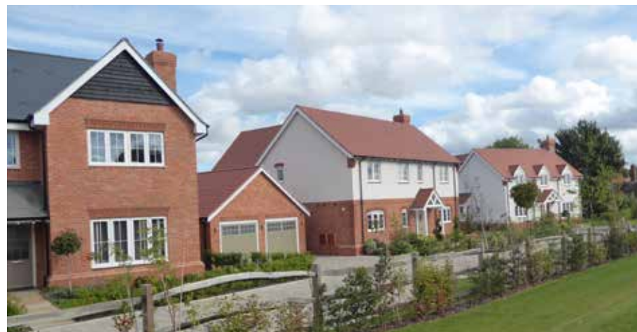
Figure 97: Modern housing on Priors Hill
