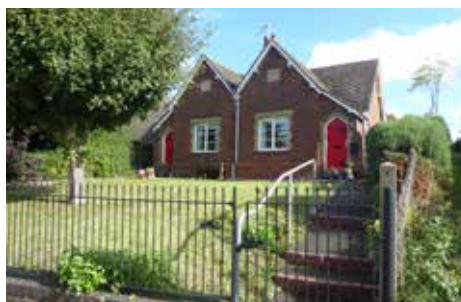
Figure 78: 19 and 21 High Street
