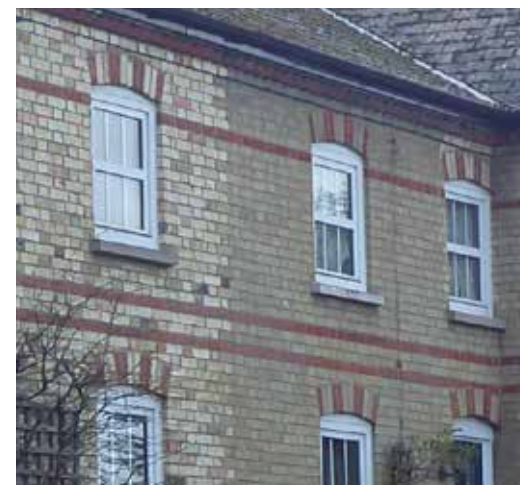
Figure 61: An example of where modern uPVC windows have been installed to replace wooden sashes
