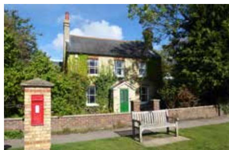
Figure 69: Open Space at Cromwell Cottage
