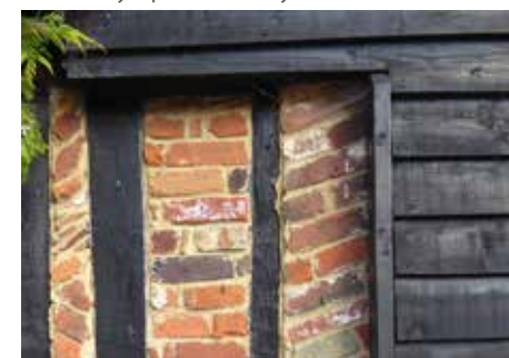
Figure 42: Example of exposed brick nogging
