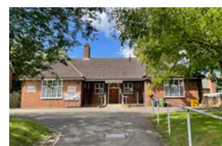
Figure 72: The Village Hall, High Street
