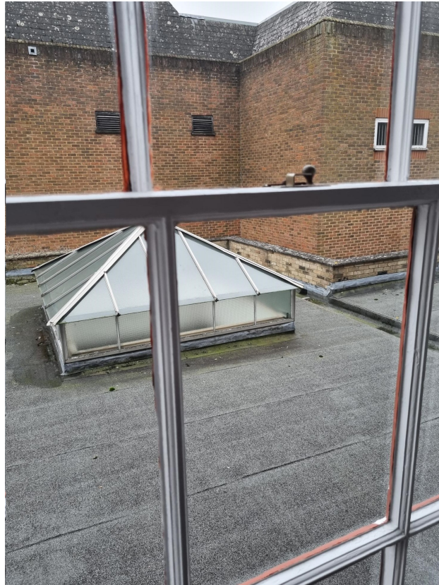
Photo taken from the first floor office window over existing flat roof rear extension
