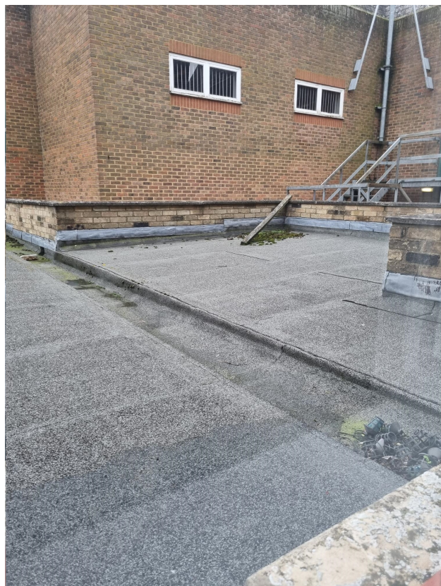
Photo taken from the half landing of principal stair case, over existing flat roof rear extension
