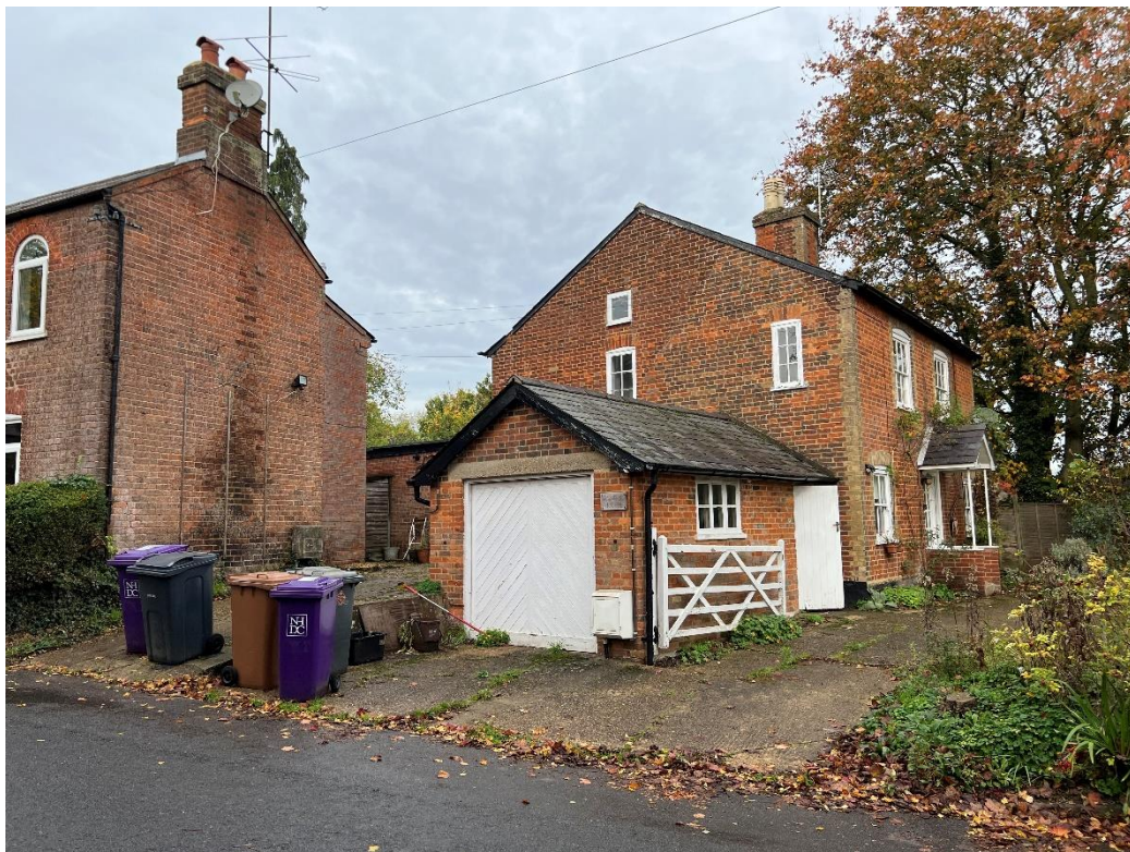
4. View of Side Elevation of Property looking from Bendish Lane – Showing location of neighbouring property 'Box Villa'
