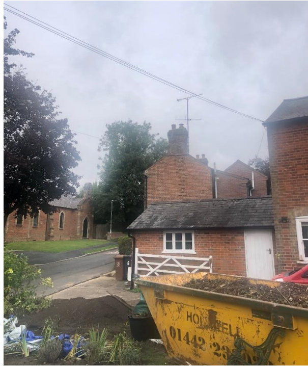
1. Current View of Front (East) Elevation from Front Garden
