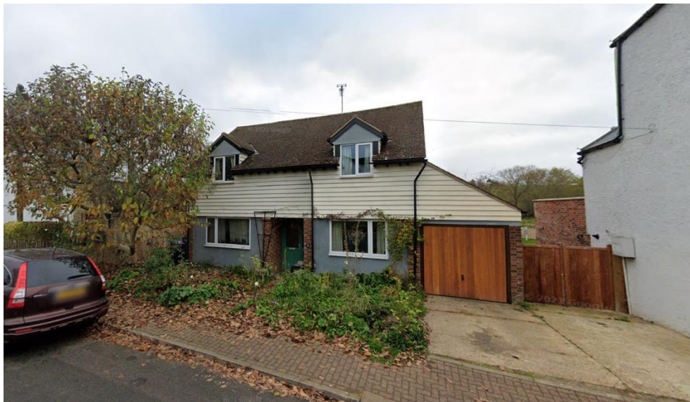
No. 26 Whitwell High Street – Demonstrating Painted Timber Weatherboarding to Front Elevation
