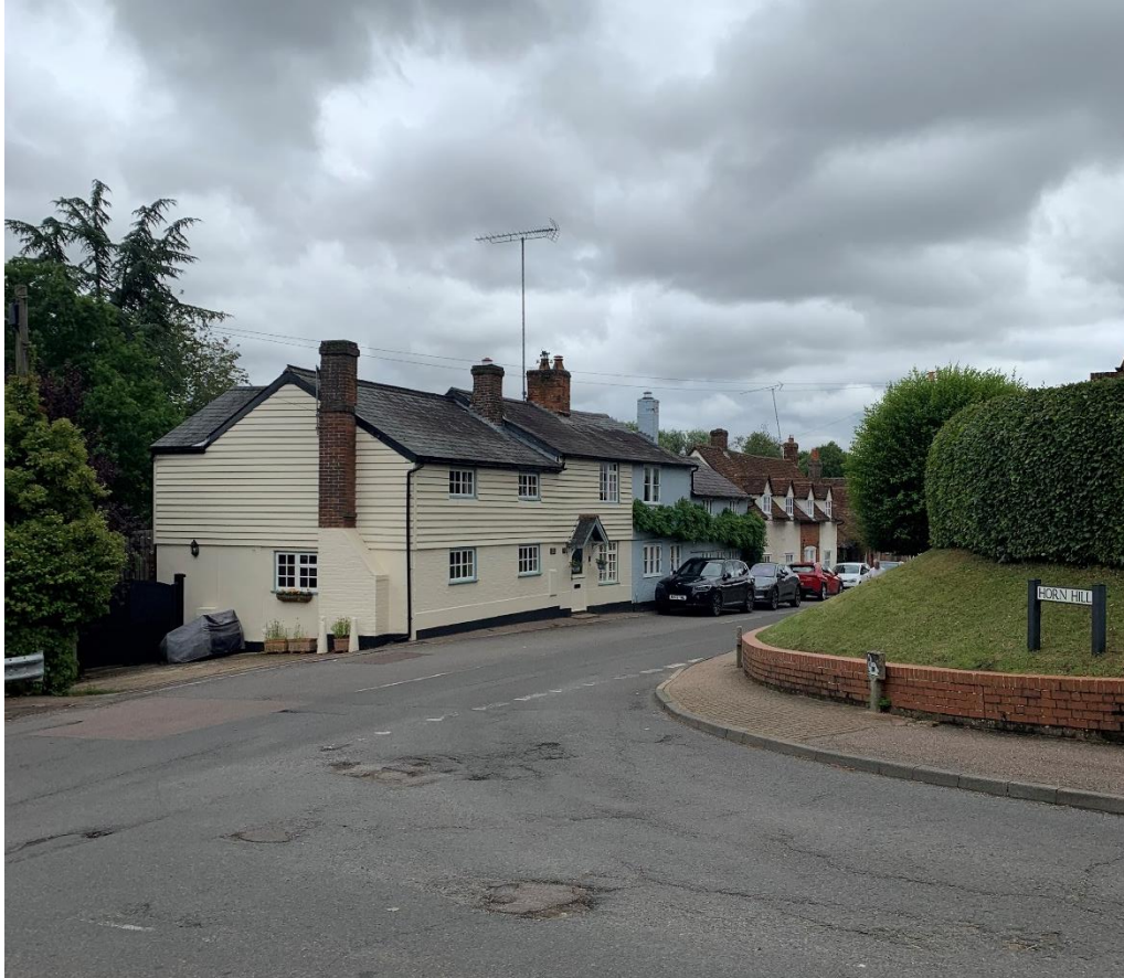
Willow Cottage, No. 76 Whitwell High Street – Demonstrating Timber Weatherboarding to First Floor Level
