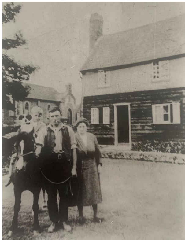
2. Historic View of Front Elevation from Front Garden (Ref St Mary's Chapel in background)
