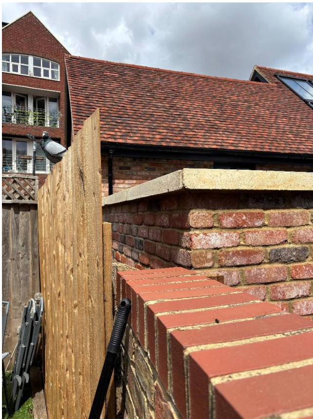
Image 1: Proximity of terrace and boundary of 1 Winch's Yard
