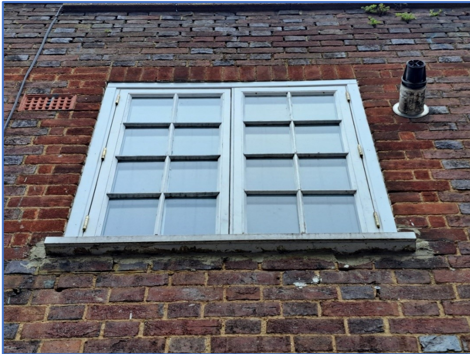
Figure 3 – Photograph of Window 7 - First floor window
