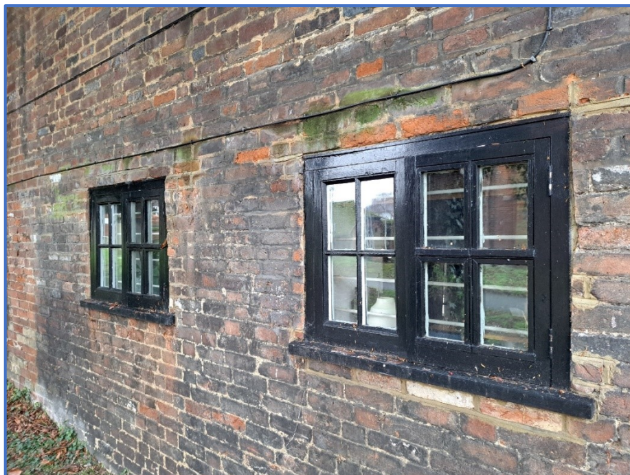
Figure 4 – Ground floor windows to side elevation
