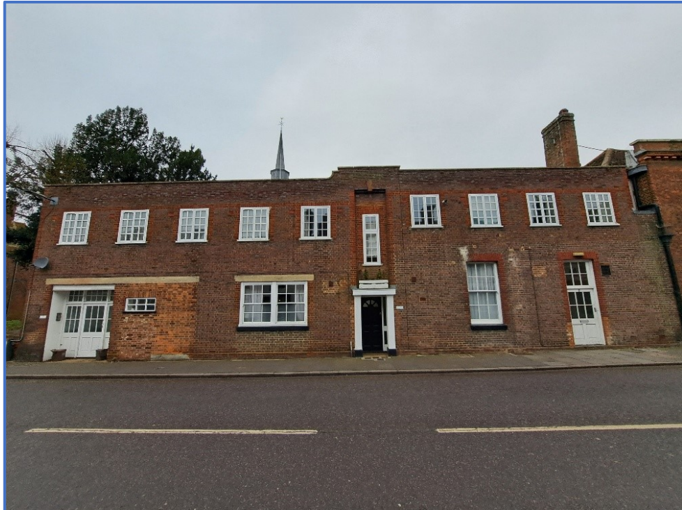
Figure 1 – The whole front elevation of Flats 1-6 Coach Yard
