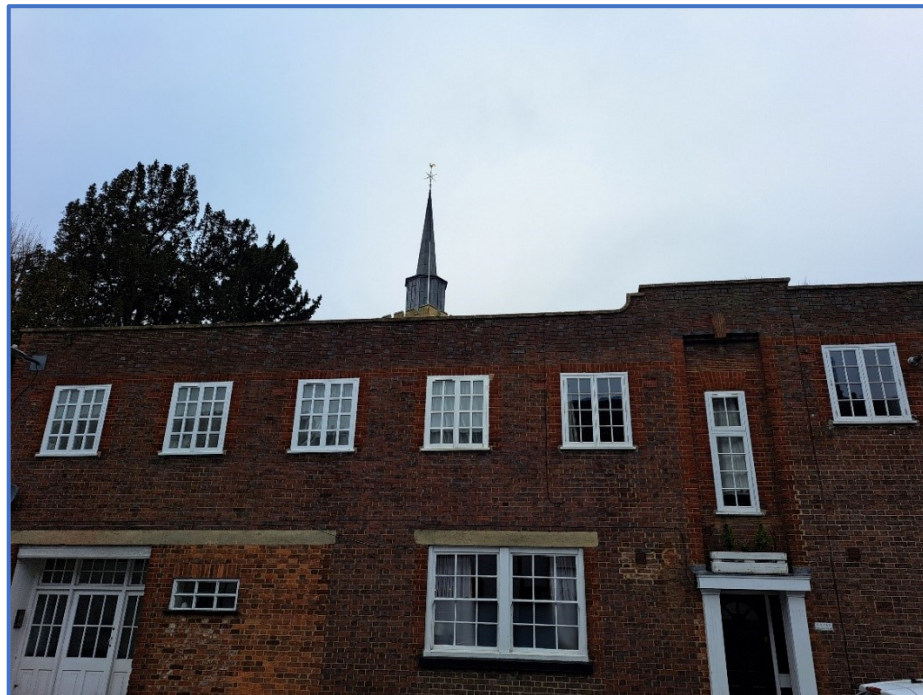
Figure 2 – First floor windows to front elevation
