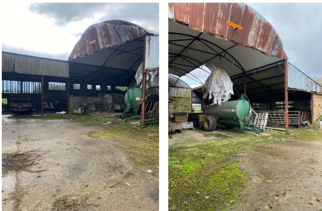
Image 1. Existing buildings at Little Manor Farm
