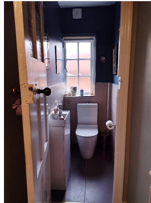
05 Existing WC viewed from landing.
