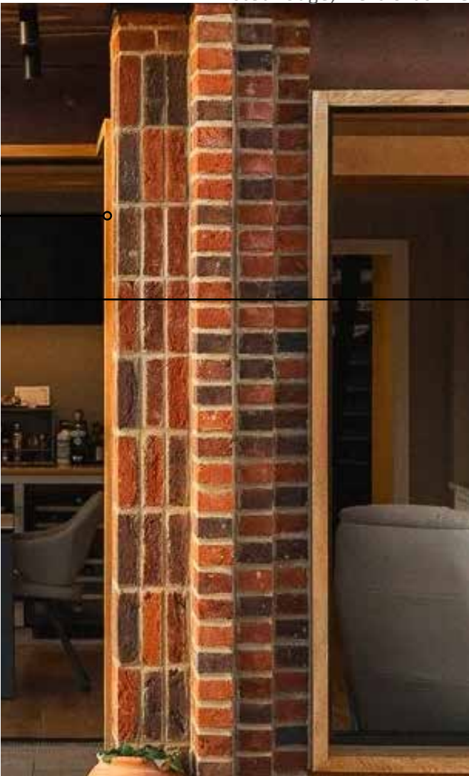
Multi-tonal brick with timber window surrounds Listed lodge, Hertfordshire
