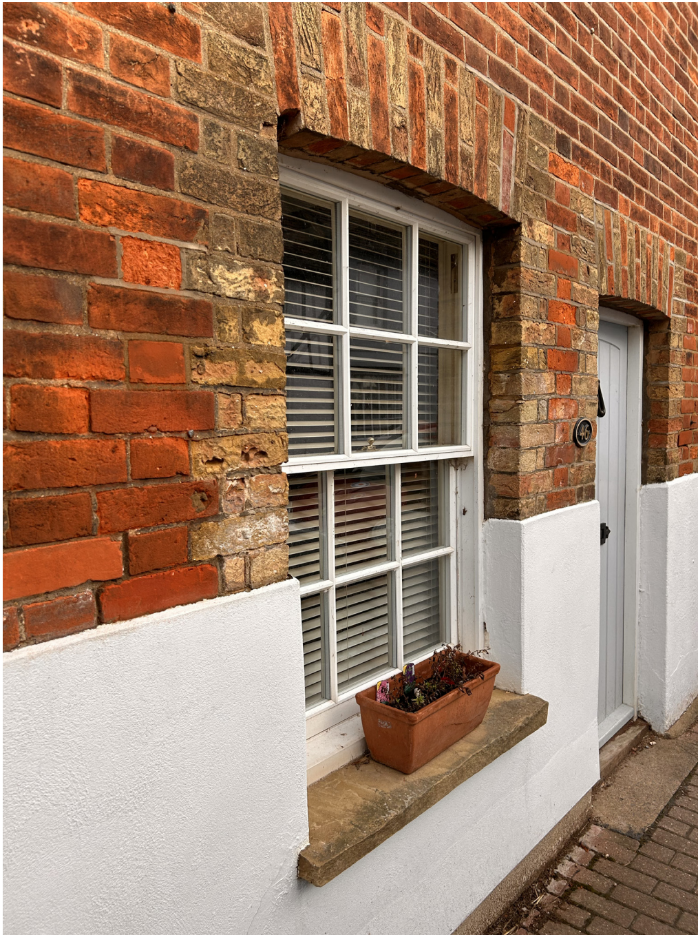
Existing neighbouring double-glazed sash window
