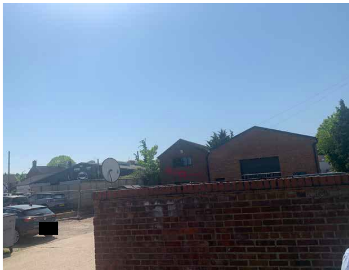
Location: West adjacent to site Building type: (including Detached/Semi/Terraced/Flats): Detached Light Industrial No. Storeys: 2 Buildings materials: Brick Parking: Off Street
