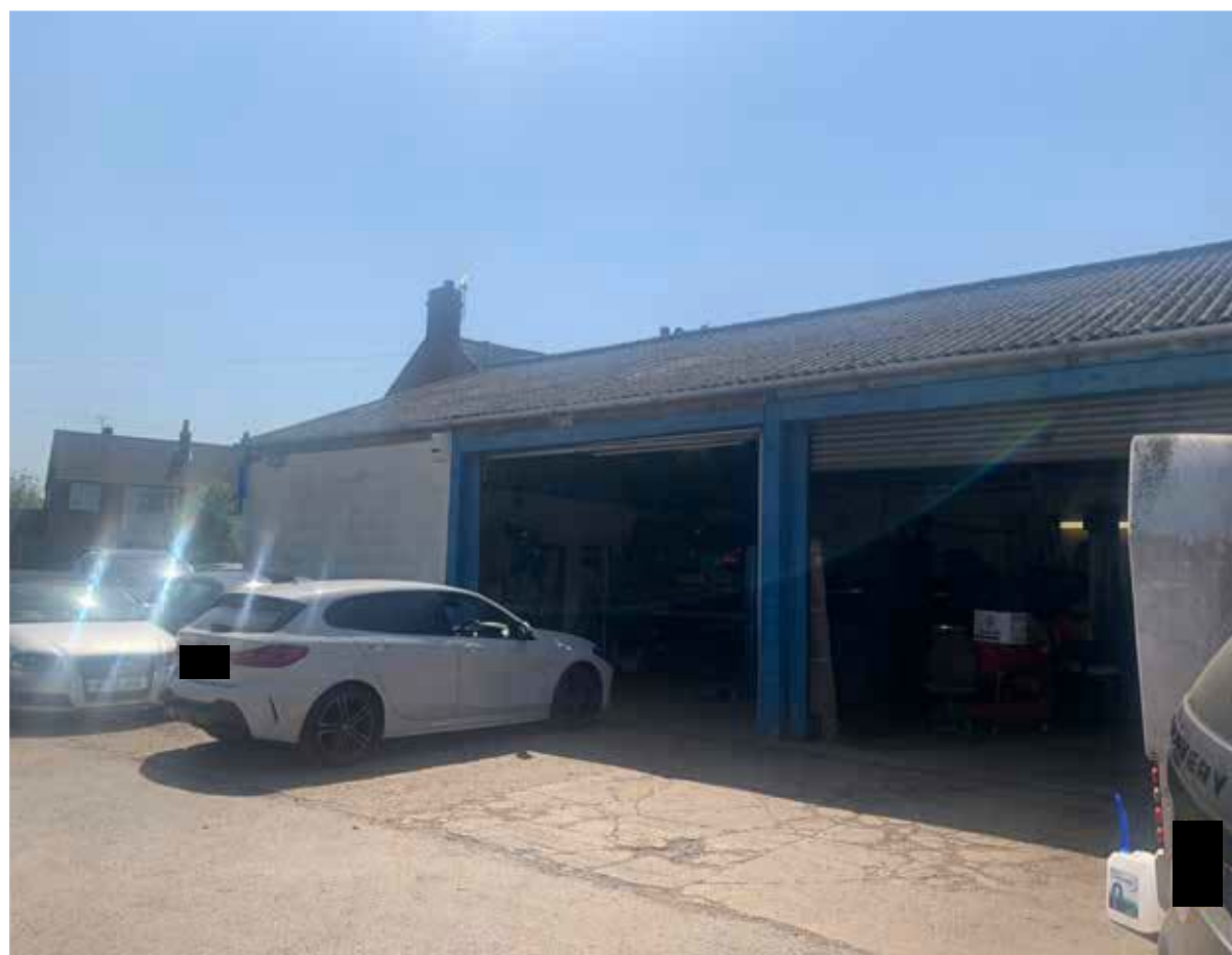
Location: South adjacent to site Building type: (including Detached/Semi/Terraced/Flats): Detached Light Industrial No. Storeys: 1 Buildings materials: Brick, Metal Cladding Parking: Off Street
