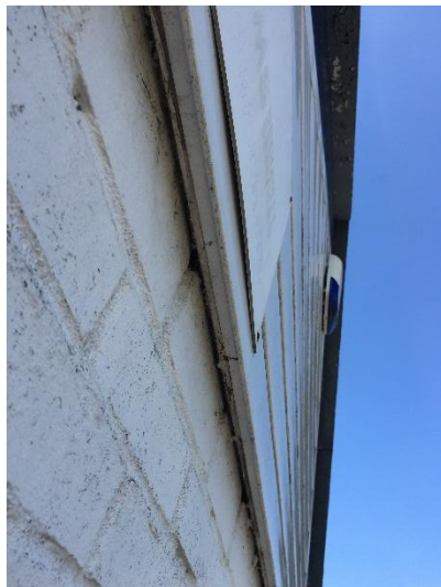
Photo 11: Gap behind uPVC weatherboarding on northern elevation of B6
