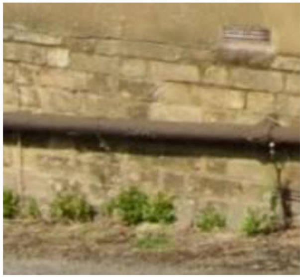
Facing Brickwork: (buff)
