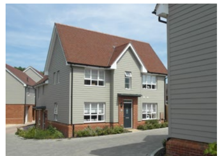
WEATHERBOARDING MATERIALS ON MAIN ELEVATIONS IN OAKHURST PLACE ©BDW
