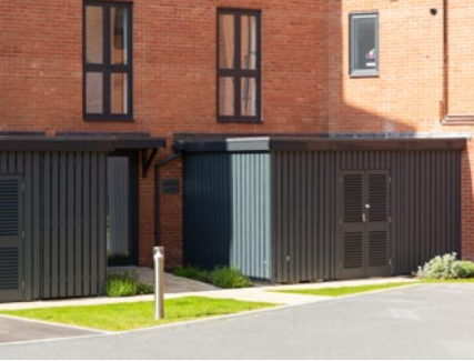
EXTERNAL BIKE STORAGE FOR FLATS LANDMARK SQUARE, WOKINGHAM ©BDW
