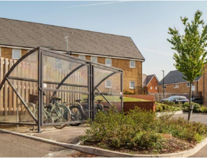
EXTERNAL BIKE STORAGE FOR FLATS CHAPEL GATE, BASINGSTOKE ©BDW
