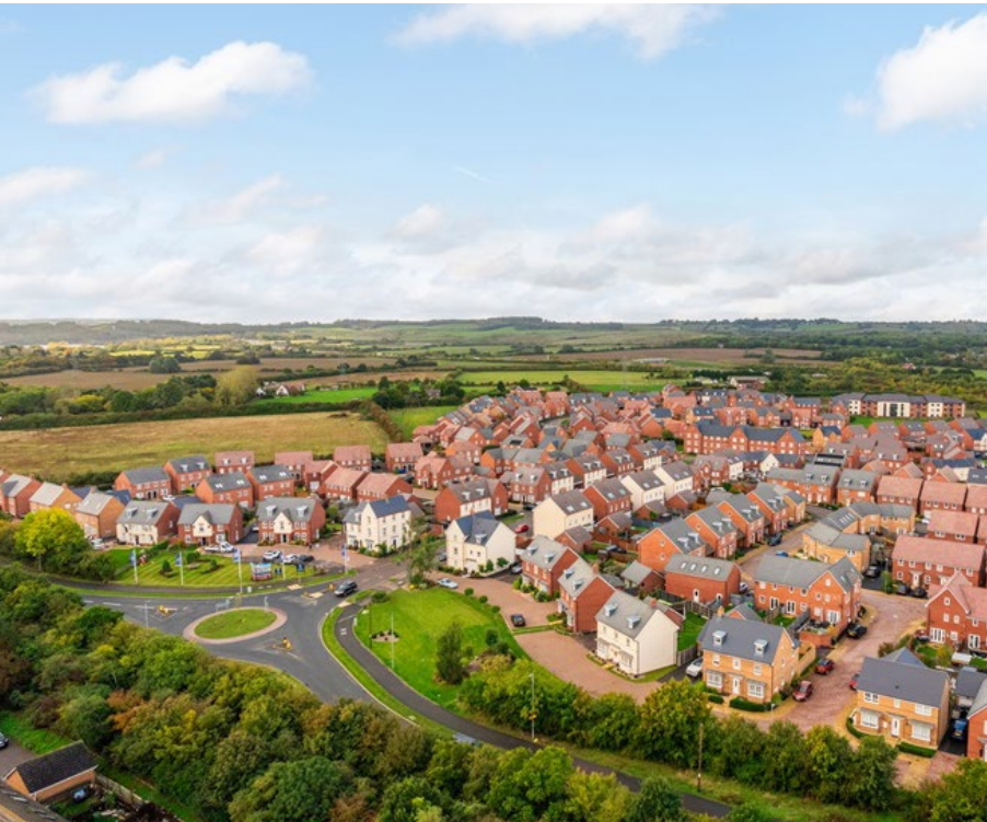
MAIN ACCESS TO THE DEVELOPMENT IN MARSTON FIELDS ©BDW
