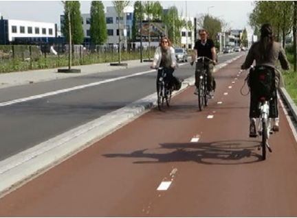
SURFACING OF SEGREGATED CYCLEWAY ©BICYCLEDUTCH
