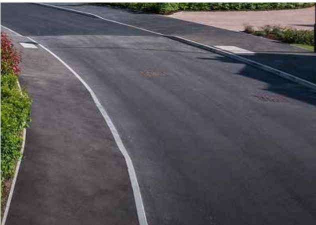
Tarmac roads and pavements
