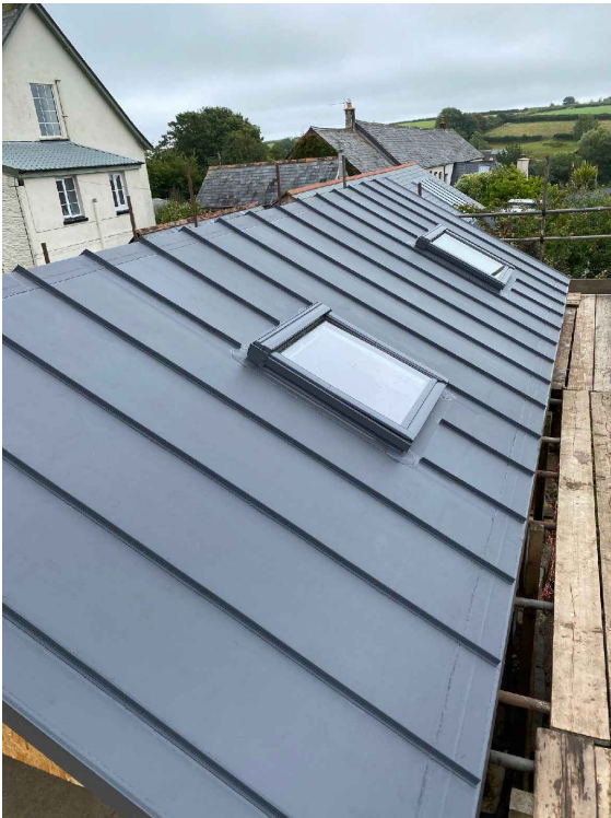
SINGLE PLY MEMBRANE STANDING SEAM ROOF
