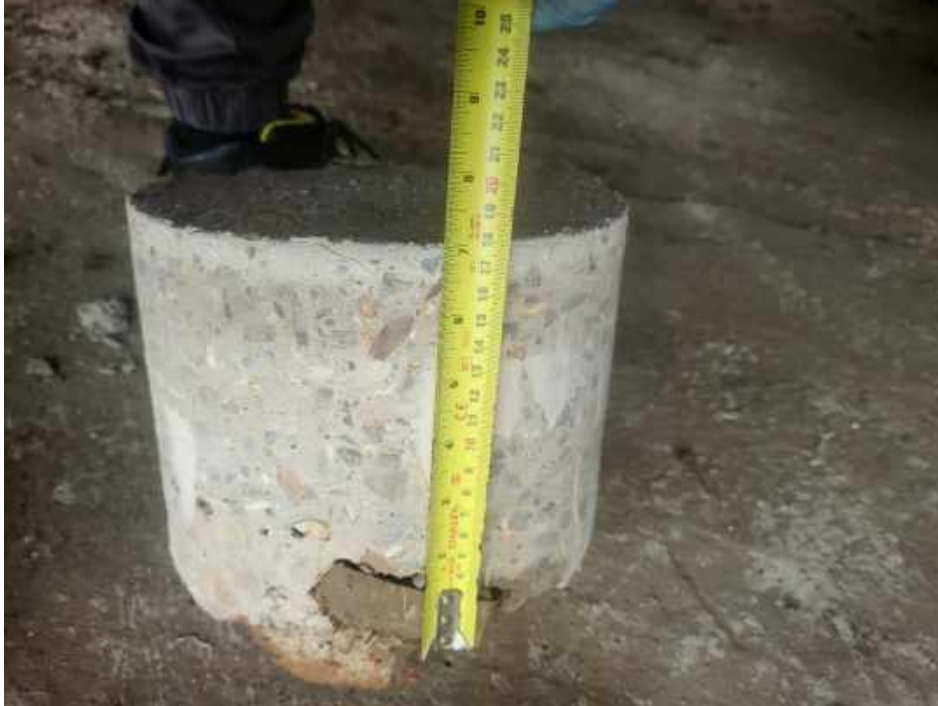
Photo 5 – Concrete Core from inside the barn (BH1)
