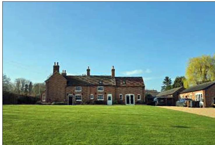
Plate 10: Southeast elevation of Pound Farmhouse, facing northeast © TAS Architects
