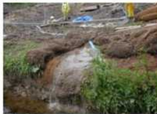
Deployed to treat muddy excavation water
