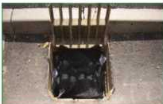
5. Close gully grid.
