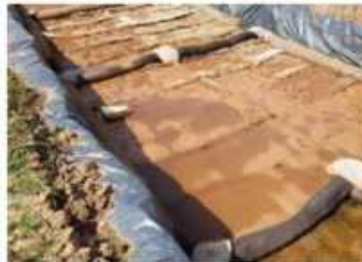
Deployed in Silt Capture Channels with Silt Wattles
